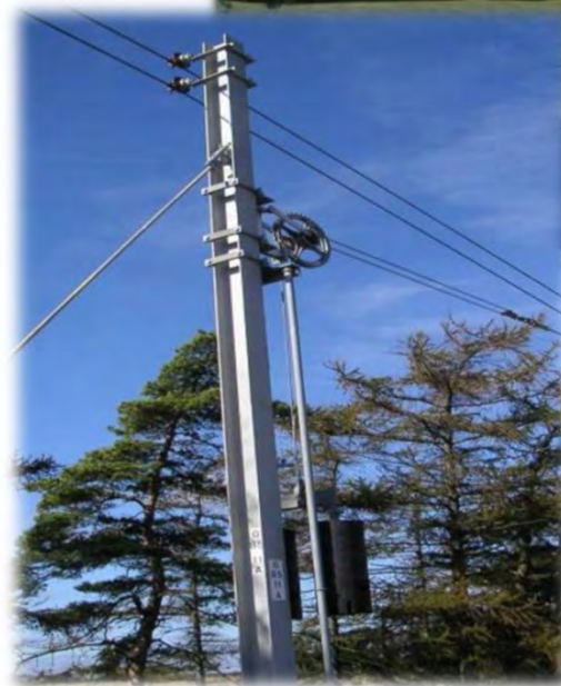
Traditional Balance Weight Anchor
