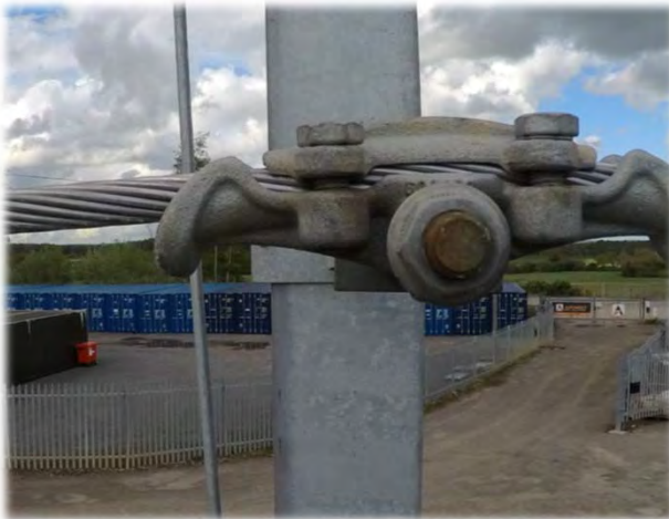
Camera on the pole
