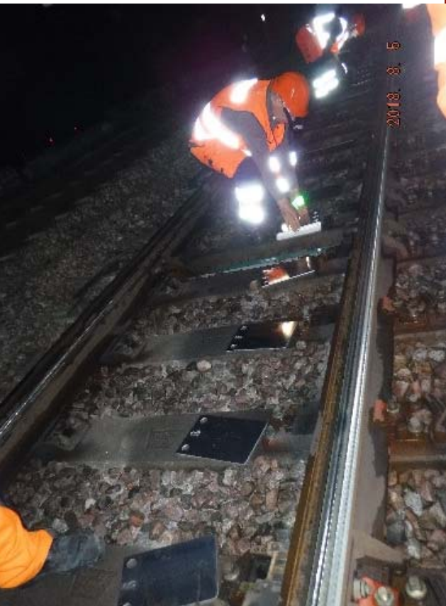
Switch rail height correction
