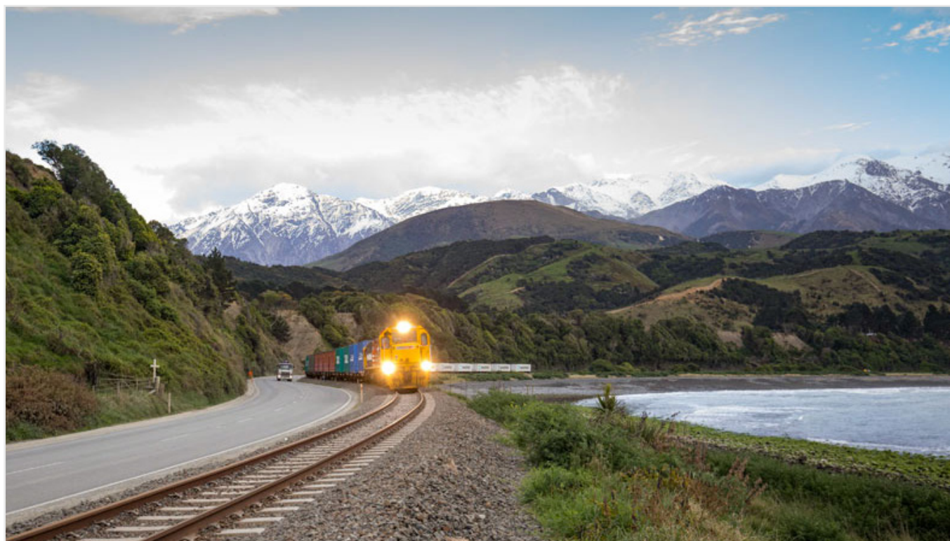
Image 11: KiwiRail freight train on the rebuilt North Main line. Photo courtesy of KiwiRail
