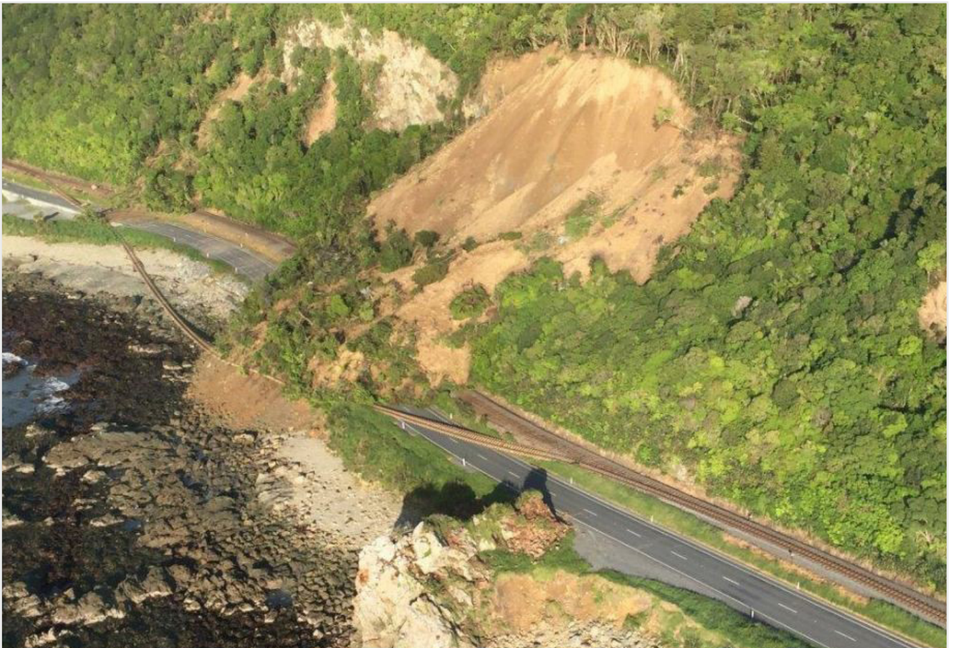
Image 4: One of the numerous, devastating landslips that buried State Highway 1 and the North Main line between Kaikoura and Blenheim. Photo courtesy of Tim Burt
