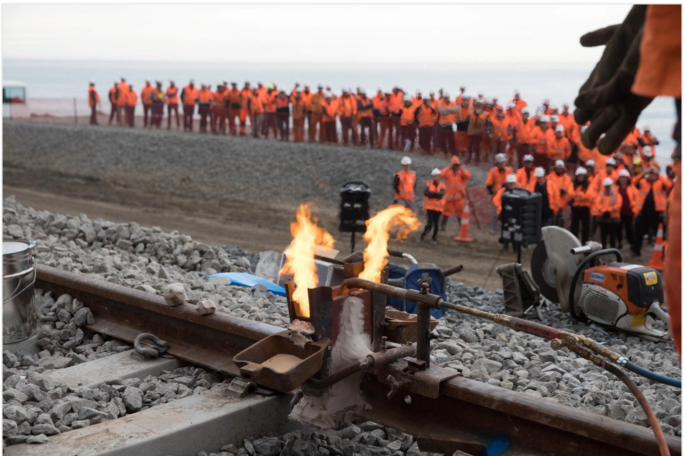
Image 10: The final Thermit rail weld at Kaikoura . Photo courtesy of KiwiRail
