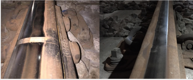
Figure 2: Rail burn beyond a 12mm T-piece
