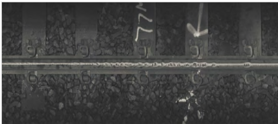
Figure 9: PLPR imagery showing multiple rail surface defects
