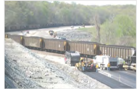
Figure 11: Open track applications; In-service asphalt paved track used for elevated BNSF/UP grade-separated track through Wichita, Kansas, placed in 2009, (top) and construction of asphalt paved track for re-alignment and triple tracking of BNSF/UP mainline east of Kansas City Near Eton, Missouri, placed in 2010, (bottom).
