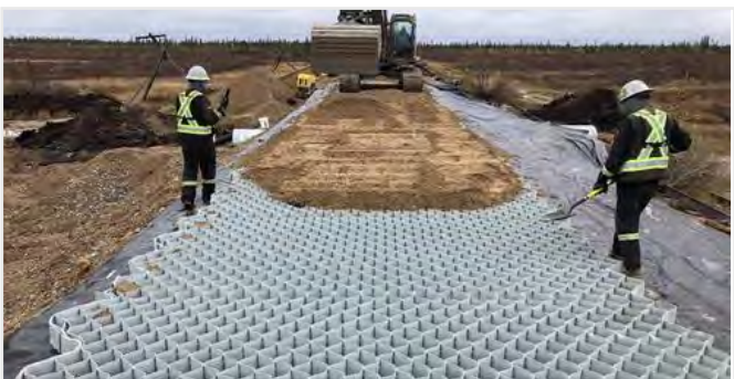
Typical culvert works and Geocell earthworks stabilisation. Images: Paradox Access Inc.
