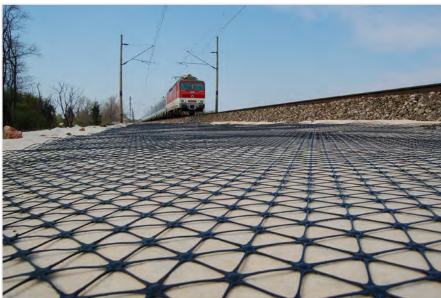
Figure 2: The new design method has been tested during full-scale field trials on live freight and passenger lines.
