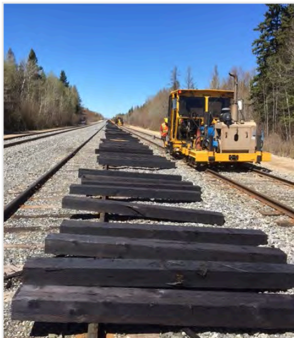
Resleeper in progress. Image: Arctic Gateway Inc.
