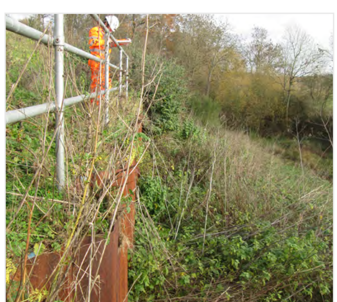
D) 50m 73 to 75ch Up. Recent photo along sheet pile wall showing good horizontal alignment.
