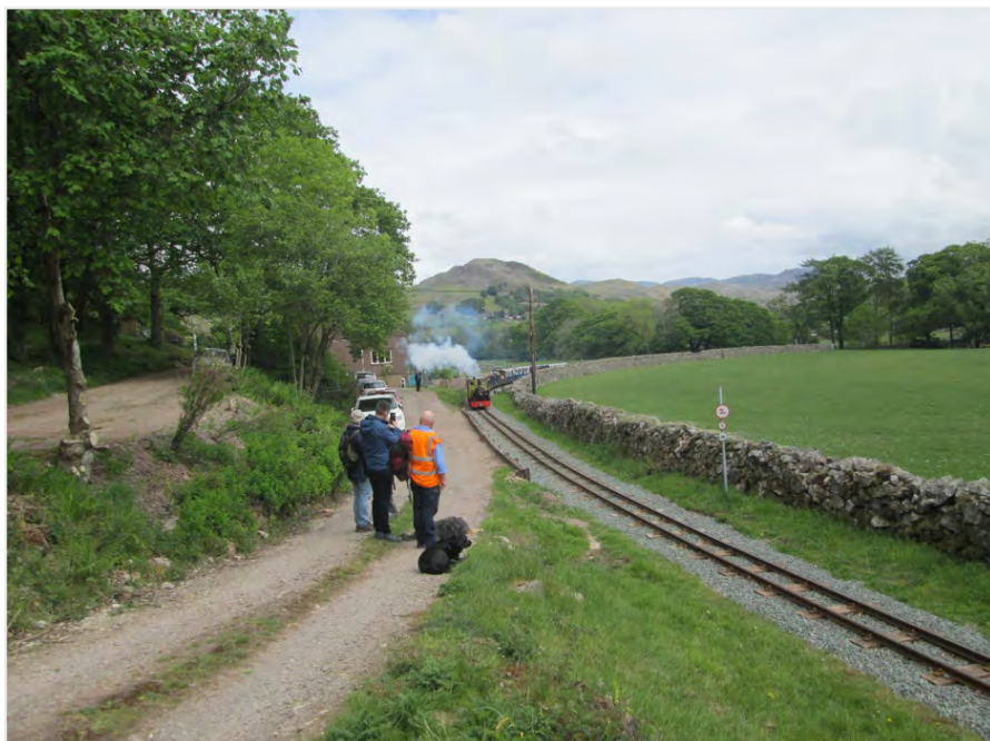
Lancaster Barrow and Carlisle Section Photograph 2: Dalegarth relaying site and sleeper retaining wall
