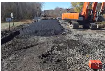
Figure 7: Turnout renewals; No. 20 equilateral concrete tie turnout on a NS mainline at Grey Eagle, West Virginia placed in 2012 and essentially maintenance free (top) and asphalt underlayment being recently placed prior to installing a No. 15 lateral wood tie turnout on NS mainline at Crandall, Indiana (bottom).
