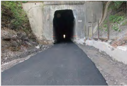
Figure 9: Tunnel floors and portal approaches; Vasper, one of three CSX mainline tunnel projects performed in the mid-1990s on mainline in East Tennessee (top) and Grey Eagle, one of three tunnels NS paved with asphalt as part of the Heartland Corridor project in 2010 near Kermit, West Virginia (bottom).
