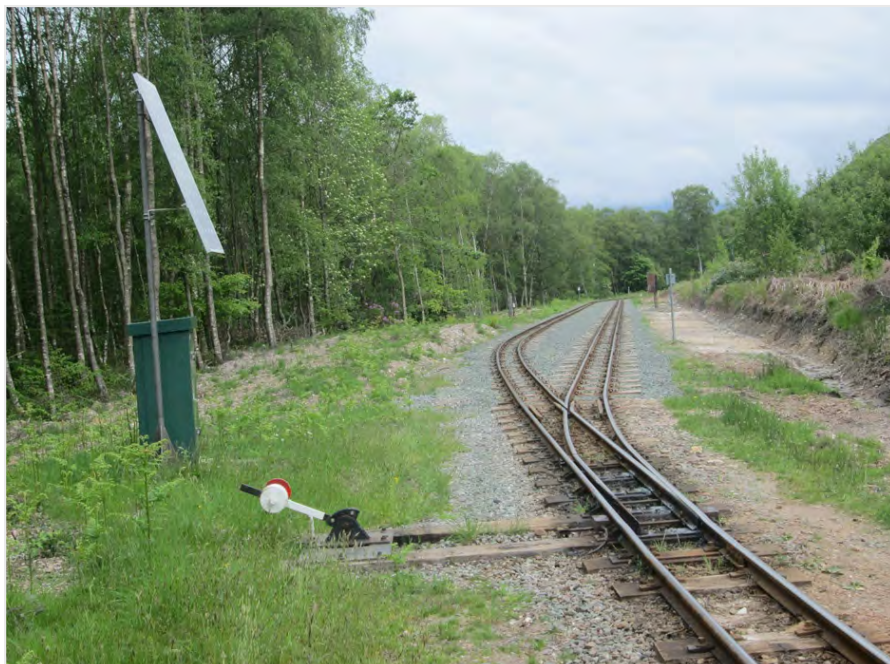
Lancaster Barrow and Carlisle Section Photograph 1: Miteside loop looking east following relaying
