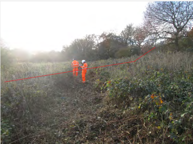
C) 50m 01 to 05ch Up. Toe berm – ash and clinker construction – possible historic stabilisation
