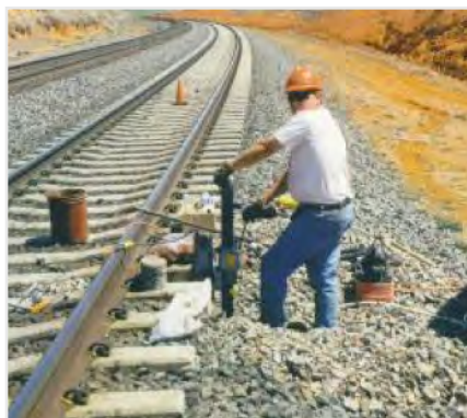
Figure 2: Core drilling asphalt, subballast, and subgrade on a CSX new bridge approach at Bridgeport, Alabama (top) and on the Burlington Northern Santa Fe Railroad (BNSF) Southern Transcon in Oklahoma (bottom).
