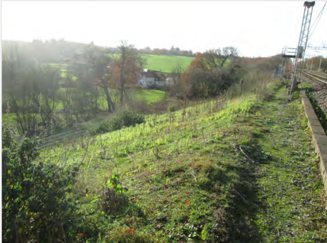
A) 49m 73 to 75ch Up. Good condition slope above existing sheet pile wall earthwork renewal
