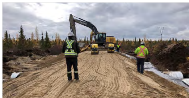
Typical culvert works and Geocell earthworks stabilisation. Images: Paradox Access Inc.
