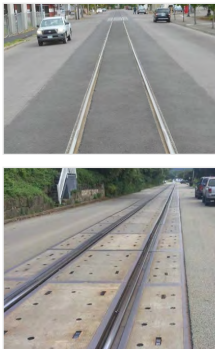
Figure 6: Middle-of-Street Crossings; Low-budget crossing on the Portland & Western Railroad in western Oregon (top) and 1000 m (3300 ft) concrete crossing on a Norfolk Southern (NS) coal line in West Brownsville, PA (bottom).
