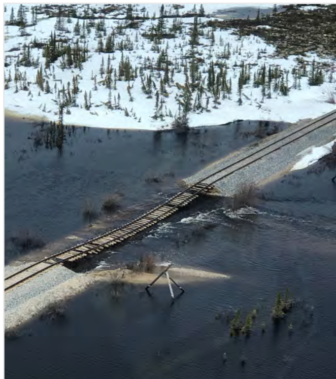
Aerial view of 200 year flooding, Manitoba (left). Typical trackbed washout (right). Images: OmniTRAX Inc.
