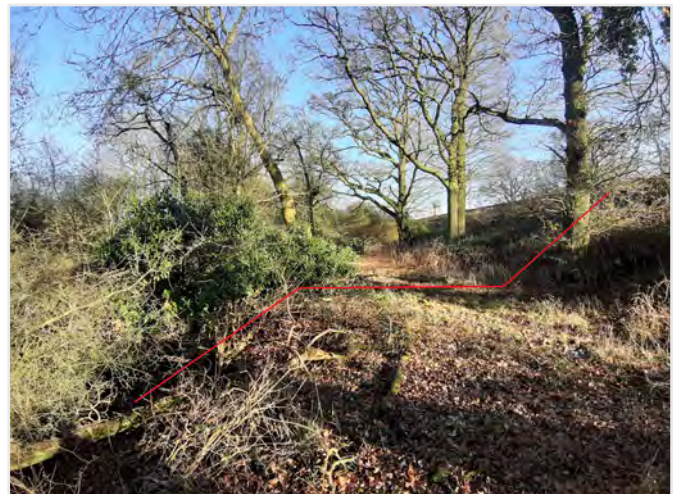
F) 50m 05 to 12ch Down. Toe berm on slope – possible historic stabilisation?
