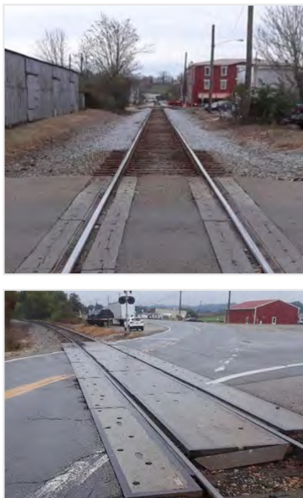
Figure 5: Railway/Highway At-Grade Crossings; CSX crossings in Cynthiana, Kentucky renewed in 1985 with the crossing surfaces only exchanged twice since then and remaining remarkably serviceable (top) and CSX crossing on WV 2 at Ashton, WV placed in 2001 with no maintenance in the 17 years and still as smooth as when it was installed (bottom).
