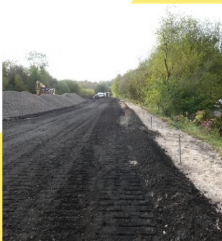
New track formation and haul road prepared
