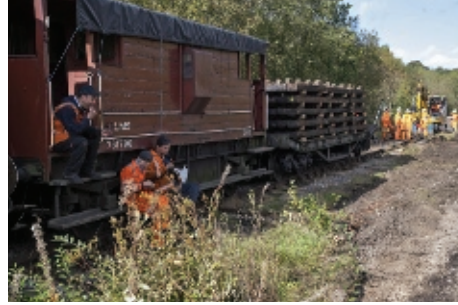
Materials train on site; wagon conveying chaired sleepers in groups of four
