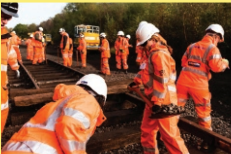
Teams distributing and boxing in ballast manually
