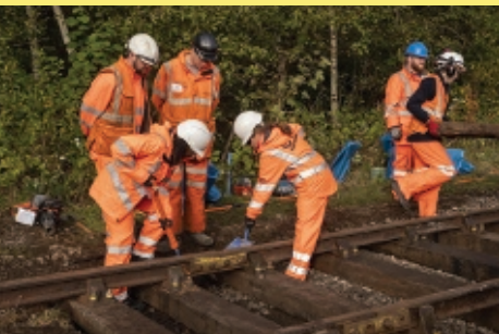
Team members manually packing run in sleepers prior to passage of materials train
