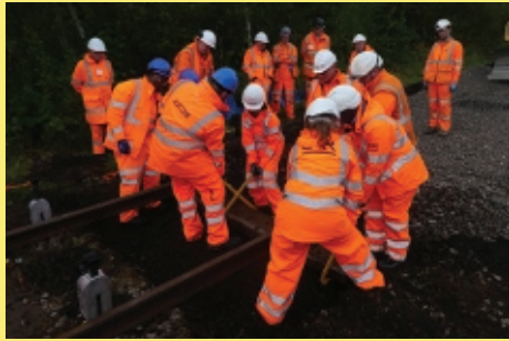
Manual sleeper threading by team members
