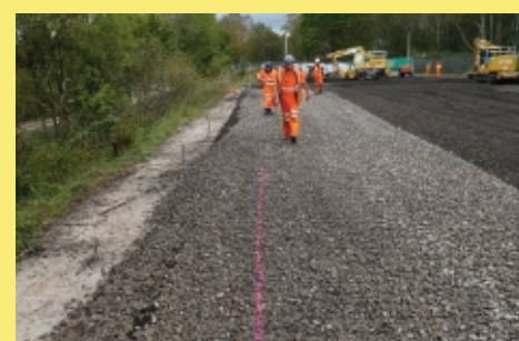
Prepared ballast bed ready for track laying
