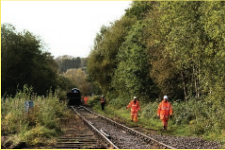
Materials train on newly laid track
