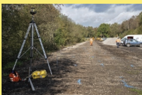
Prepared ballast bed ready for track laying
