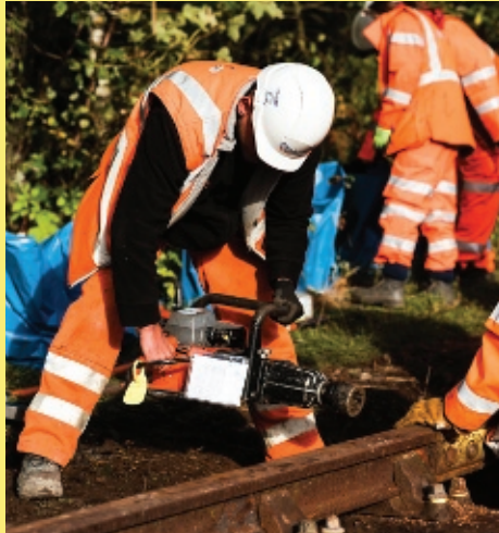
Tightening fish bolts utilising an impact wrench, supervised by Cleshar trainer
