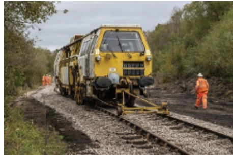
OTM tamping and lining newly laid track
