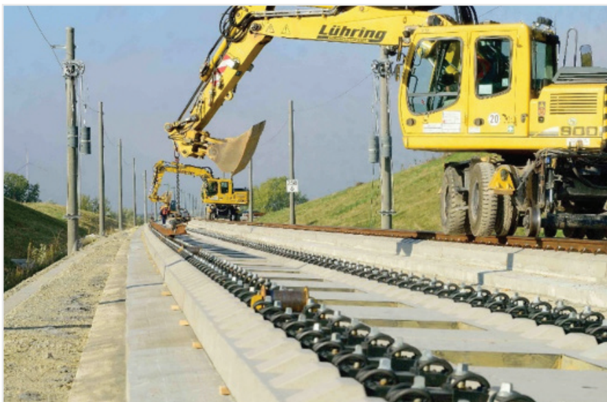
Figure 2: Rail installation on slabs.
