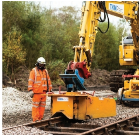
RRV with ballast profiling tool attached
