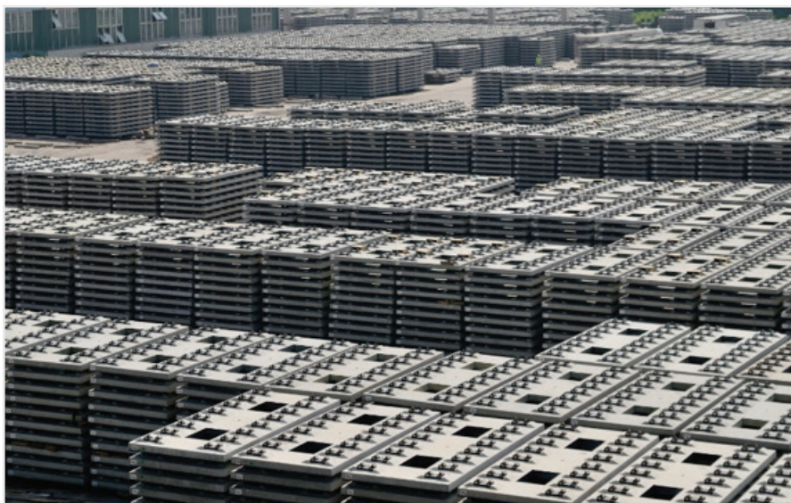
Figure 8 Storage facility for track slabs. Size of the laydown area depends on the project logistics and delivery programme.
