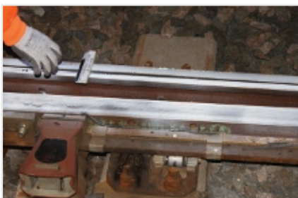
Figures 12: Commissioning tests
