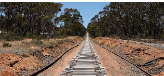
Image 4: New Pan concrete sleepers laid out on graded formation ready for rail installation (photo: WCCJB).
