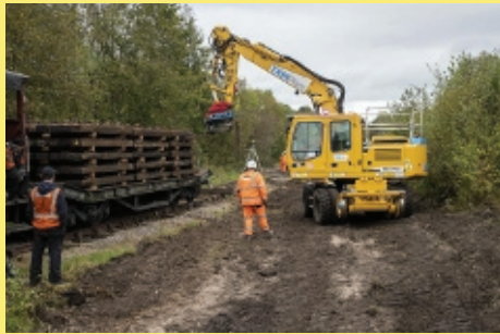
OTP with fork attachment preparing to unload sleepers from wagon in groups of four
