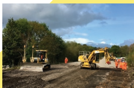
OTP D41 laser guided dozer preparing ballast bed
