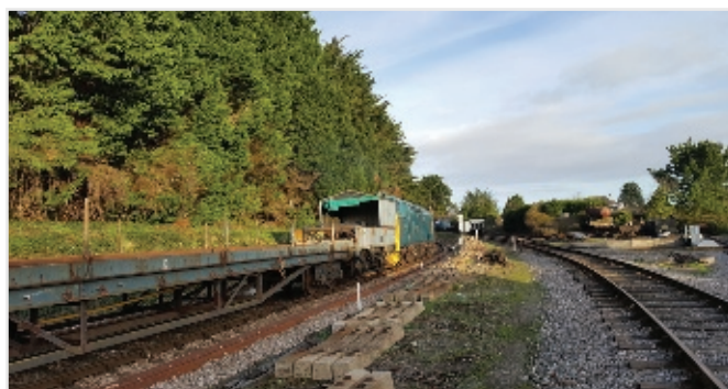
Image 2: Winch and roller set, a steel wire pulls the rails up on to the wagon and removed from site.
