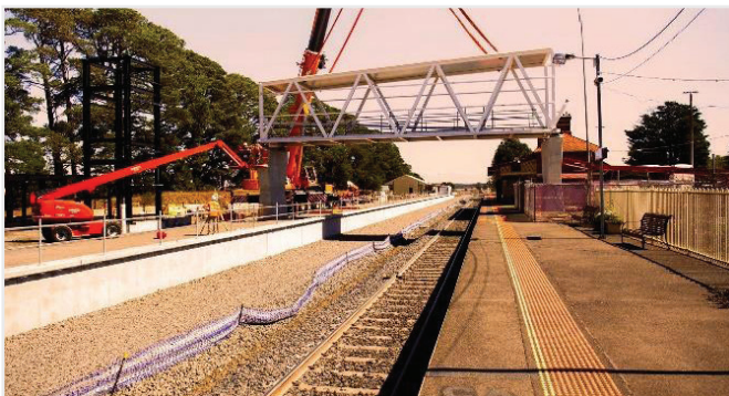
Image 10: New station platforms and footbridge
