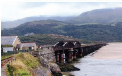
Barmouth viaduct after the rain, 28 August 2019. 100 milepost at centre left, with metric speed indicator, 35km/h near toll house (photo by Robert Hyett).
