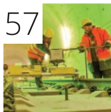
Overcoming logistic challenges when building large scale slab track railway projects
