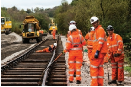
Teams manually fine aligning track
