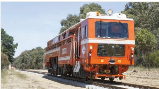
Image 5: MartinusRail Plasser 09-32 CAT on the newly re-laid standard gauge Maryborough line (image: WCCMR).
