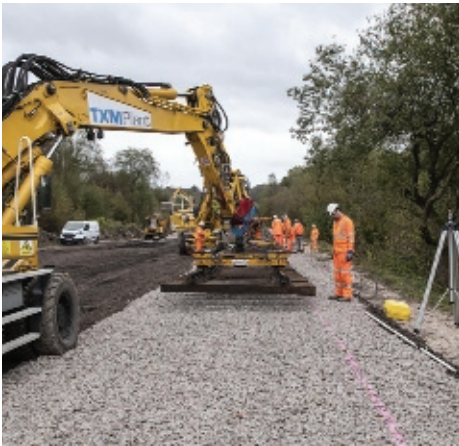
OTP in tandem placing 18.3 m track panel to design position
