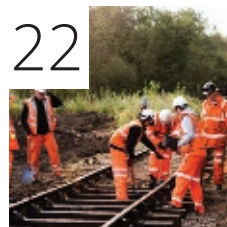
Practical trackwork challenge Churnet Valley Railway
