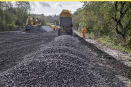
Hydrema dumper unloading trackbed ballast
