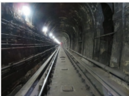
Figure 2: Rotherhithe end. The short section of unrestored tunnel.
