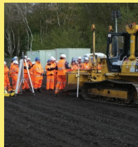
Track alignment and longitudinal level pegs set by TfL survey & design team
