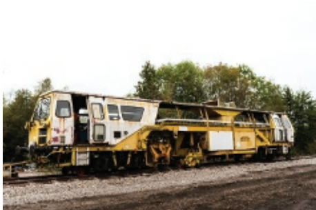
Tamping and lining newly laid track
