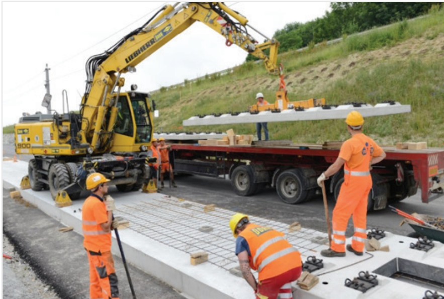
Figure 1: Slabs are transported to the construction site and laid in track with an already high precision of \pm 0.5 cm. This reduces the amount of adjustment work necessary to achieve the final precise track position.
