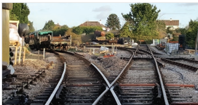
Image 1: First set of rails removed.
