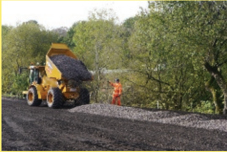
Hydrema dumper unloading trackbed ballast
