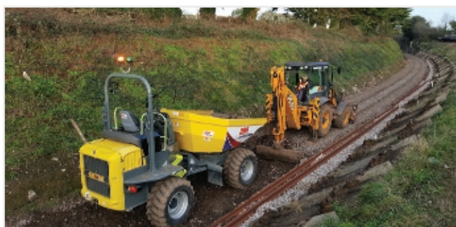
Image 3: Bottom ballast and spoil being loaded and removed.
