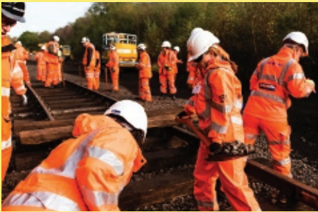
Teams distributing and boxing in ballast manually
