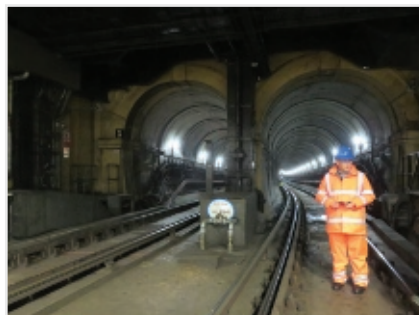
Figure 5: Twin arch design, Wrapping Station end.
