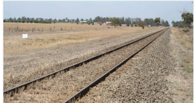
Image 1: Existing (typical) track conditions Geelong to Ballarat line, 1600 mm / 5 ft 3 in gauge (photo: WCCMW).
