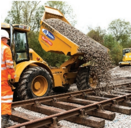
Hydrema dumper side tipping boxing in ballast
