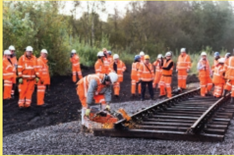
Cleshar operative using rail saw
