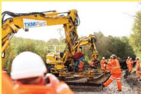
OTP in tandem for lifting, carrying and placing 18.3 m track panels
