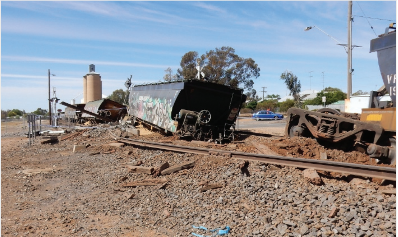
Image 7: 2015 derailed grain train at Ouyen, Victoria due to excessive CWR compression and rail creep at a fixed level crossing (photo: Transport Safety (Vic)).
