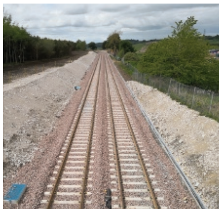
A21 redoubling (photos by R McCafferty)
