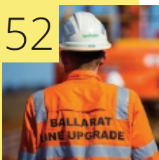
Ballarat line upgrade Regional rail revival in Australia
