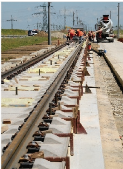
Figure 4: Grouting of the Slab Track Austria is done through tapered openings in the precast slab.
