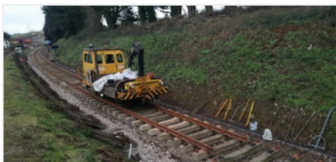
Image 5: Plasser Hopper Tram at the rail head in preparation to lift in the next batch of rails.
