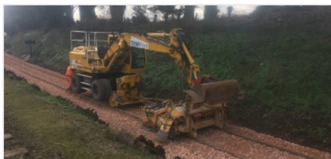
Image 7: TXM with ballast profiling brush tidying up the site.
