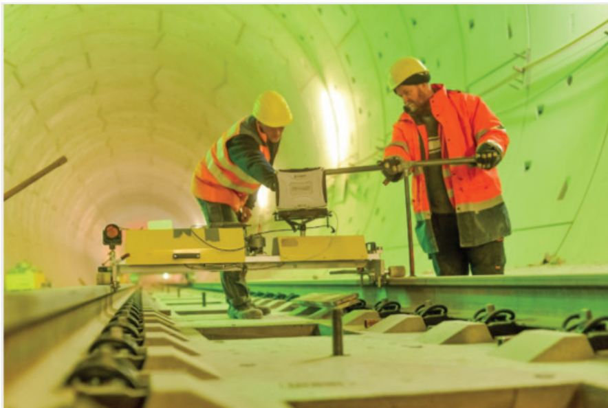
Figure 3: Survey and final adjustment of the slab track measuring from top of the rail. Alternatively, if needed, slabs can be installed without the rail, using highly precise reference points on the slab.
