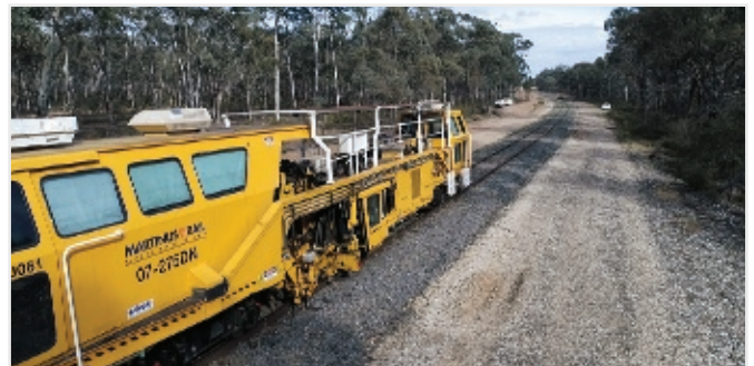
Image 3: Martinus Rail Plasser 07-275 tamper engaged upon track refurbishment works (photo: WCCMR).
