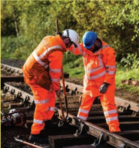
Tightening fishbolts manually
