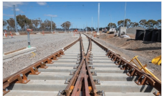
Image 9. Installation of concrete bearer switch and crossing units with flat bottom rail and Pandrol fastenings (image: RPV (Rail Projects Victoria)).
