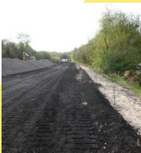
New track formation and haul road prepared
