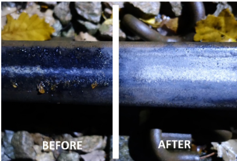
Image 2: A photograph showing where cryogenic cleaning of the 'blackened leaf layer' has stopped.
