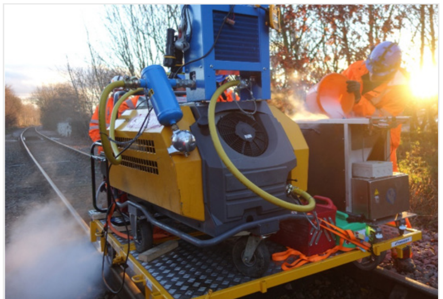
Image 1: The track trolley mounted equipment in use on a low traffic freight line in South Yorkshire.
