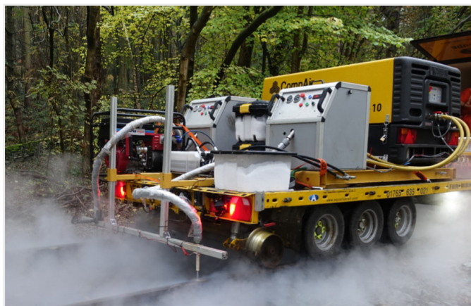
Image 5: The RRV trailer mounted cryogenic cleaning skid in operation.
