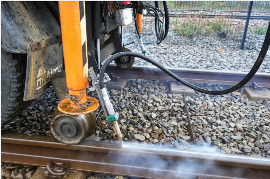
Image 3: The cryogenic cleaning system mounted on the RRV multicar at Sheffield Supertram depot, cleaning heavily oxidised track.
