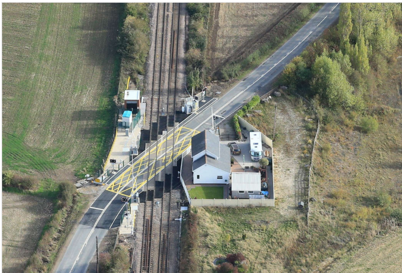
Figure 1: Aerial photograph of Commissioned Spring Lodge Level Crossing (Network Rail Route View) 3 .
