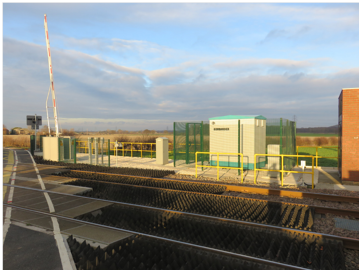
Figure 12: Photo of Commissioned Level Crossing Hut at Spring Lodge LX.
