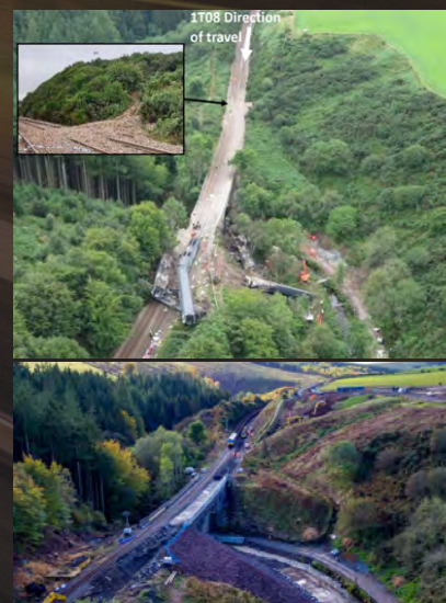
Images 5 & 6: Stonehaven Derailment August 2020, inset the washed out material and right repairs well underway in October 2020 (images courtesy Network Rail Resilience of rail infrastructure interim report to the Secretary of State for Transport following the derailment at Carmont, near Stonehaven, Andrew Haines, CEO 01-09-20; RTM)
