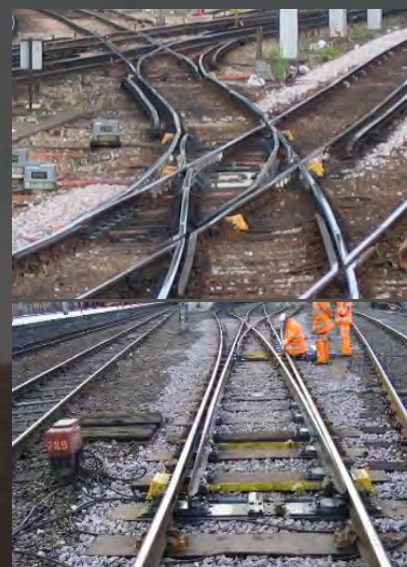
Images 3 & 4: Switches and Crossing refurbishment before and after (images by Dave Ratledge and Roy Hickman on PWI training course)
