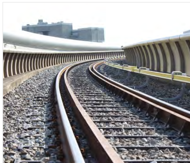
Figure 5: Polymer sleepers on a fly-over in the Netherlands, applied due to weight restrictions.
