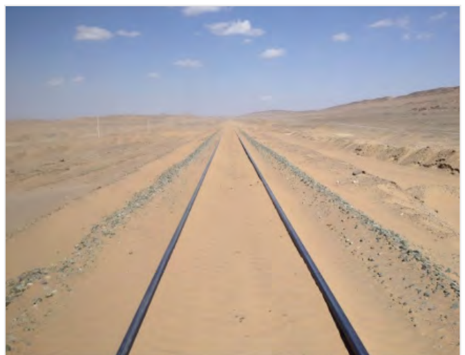
Figure 2: Ballast fouling by sand in the Yazd desert (Iran).
