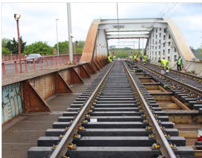
Figure 1: Polymer sleepers on a steel girder bridge in Belgium.
