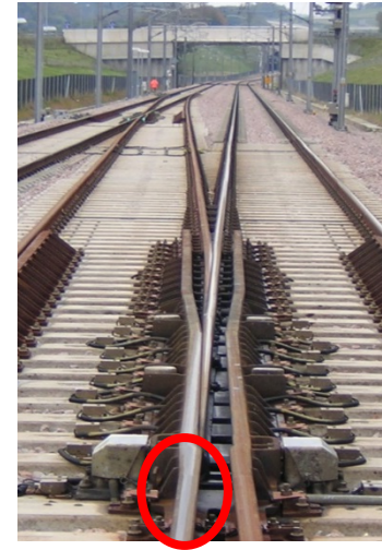
Dip in rail profile at the weld repaired section
