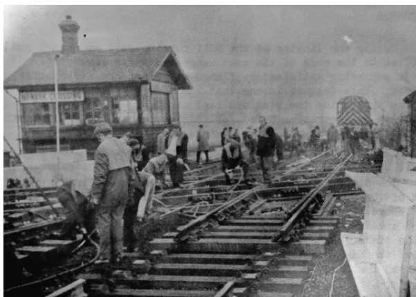
New crossings + Jarrah packing on existing timber waybeams
