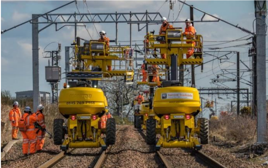
Photo: Courtesy of Network Rail West Coast
