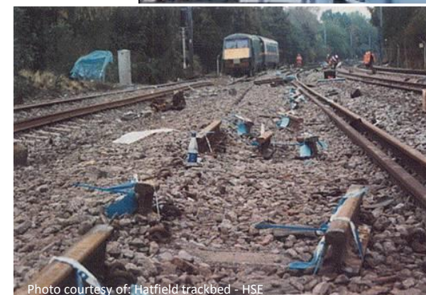
Photo courtesy of: Hatfield trackbed - HSE
