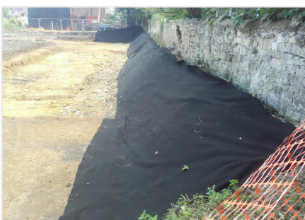
Figure 7: A root barrier installation
