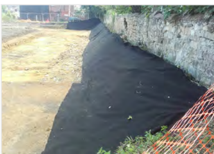
Figure 7: A root barrier installation
