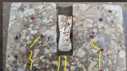
Image 6: Eastleigh derailment 28 January 2020 - The sheared pandrol housing
