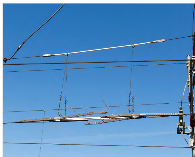
Figure 14: Arthur Flury section insulator; Rugby, UK
