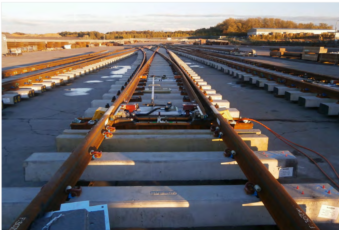
Figure 8: Battersea Pier junction assembled for NR inspection at VAE's Harworth site prior to installation, Christmas 2018
