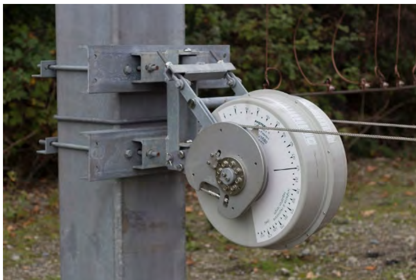
Figure 3: Pfisterer Tensorex C+ spiral torsion spring tensioner, and Tensorex spring
