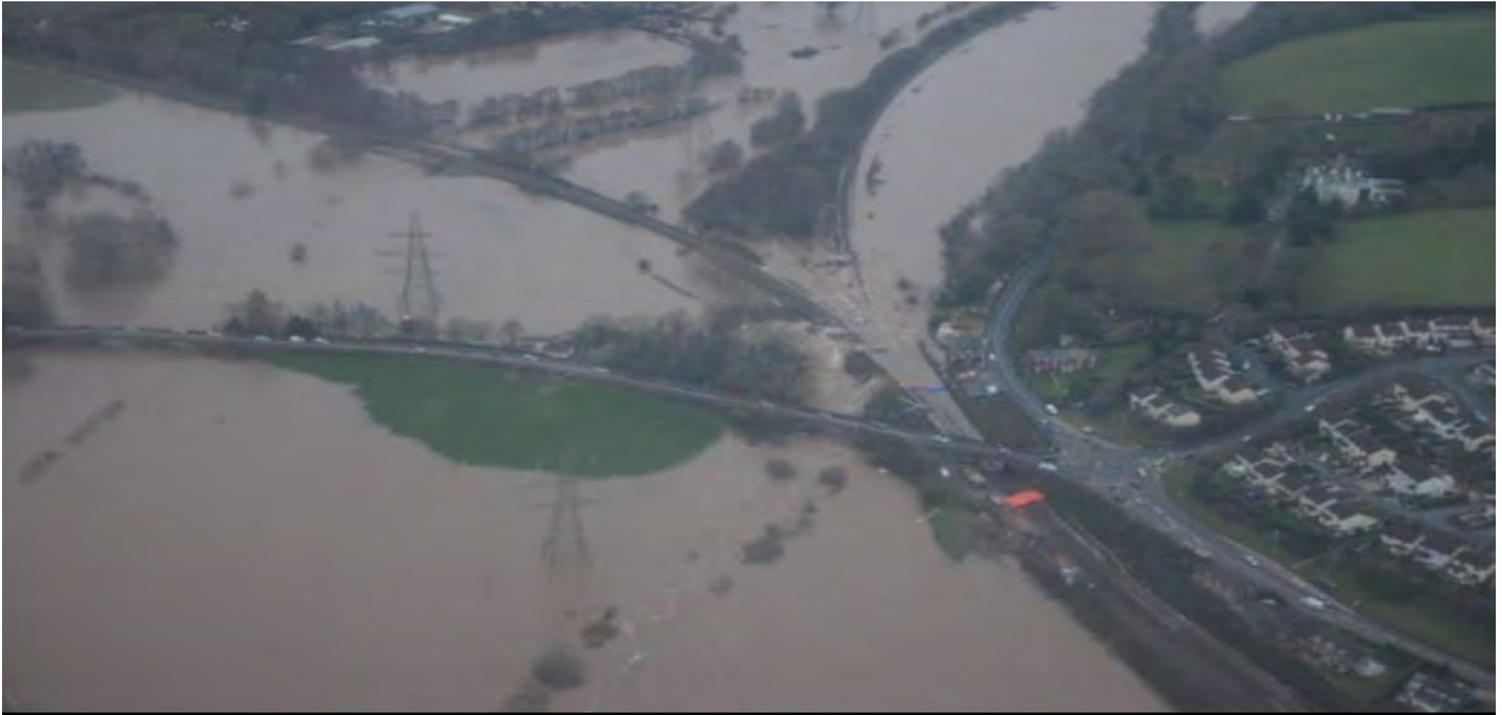
Figure 4-1: Cowley Bridge 2012 Flood Event Image source: Environment Agency Product 4 Information
