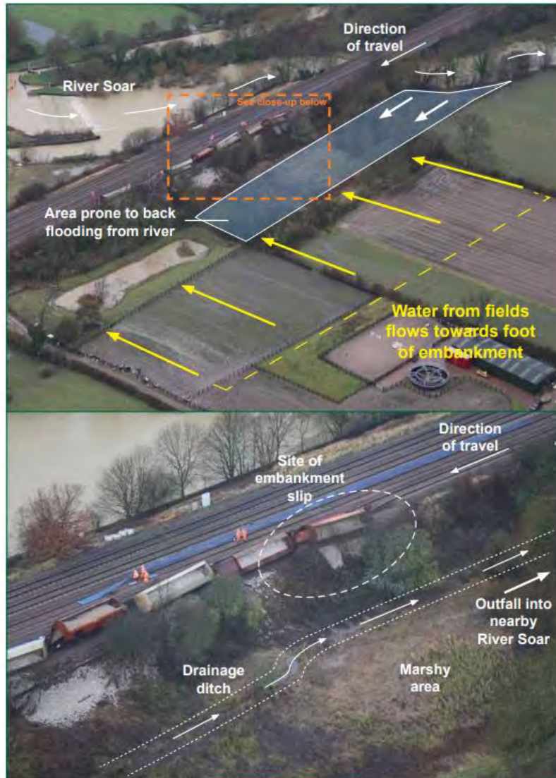
Figure 13: Drainage from the foot of the embankment to the River Soar (photographs courtesy of Network Rail)
