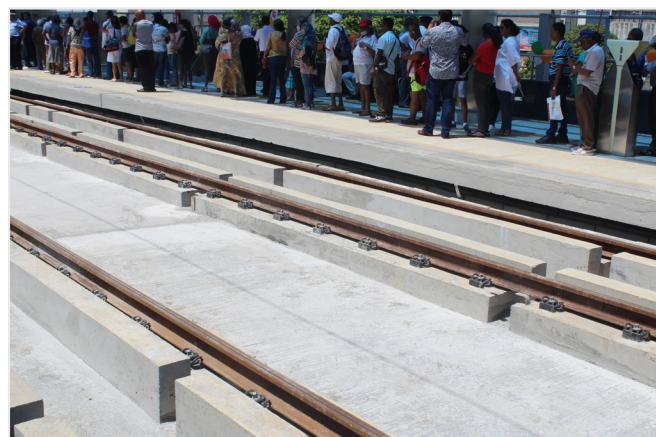
Figure 4: Track construction used on elevated sections.
