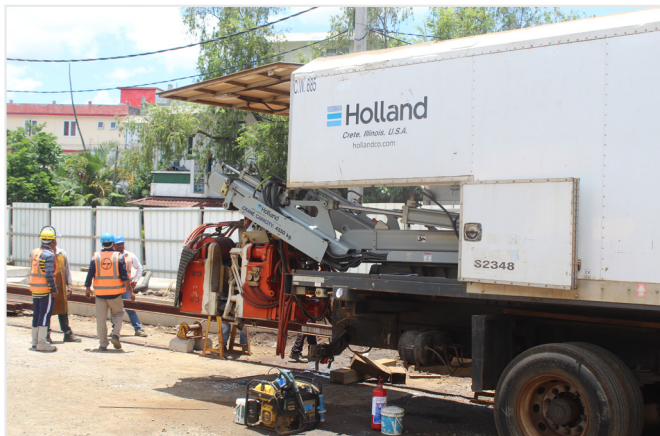
Figure 5: Portable flash butt welding machine and road mounted generator van.
