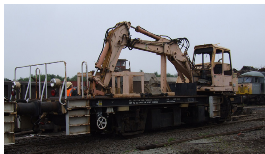
Plasser EPV 360 Atlas excavator
