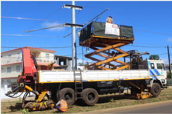
Figure 13: Installation of overhead line using a specialised road-rail lorry.
