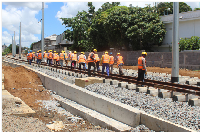
Figure 7: Final manual positioning of rails.
