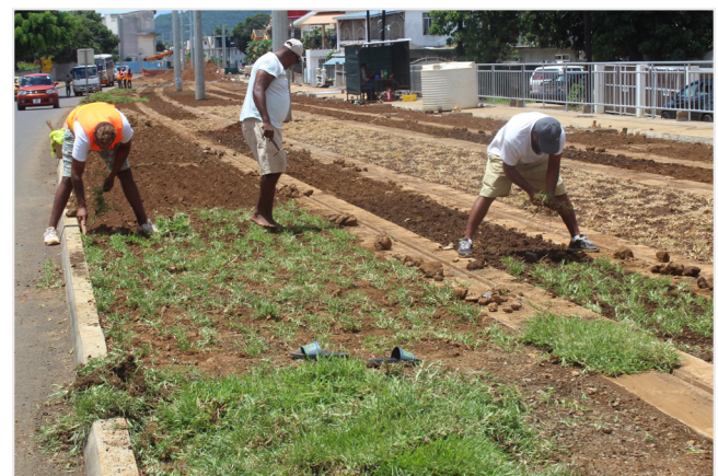
Figure 10: Grass installation adjacent to public road sections.
