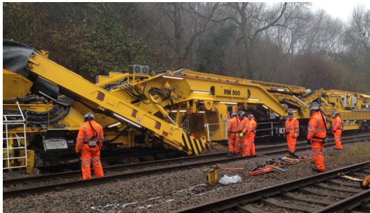
Network Rail's High Output Ballast Cleaning System
