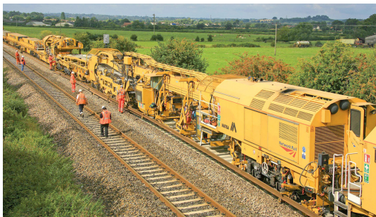
Track Renewal Train
