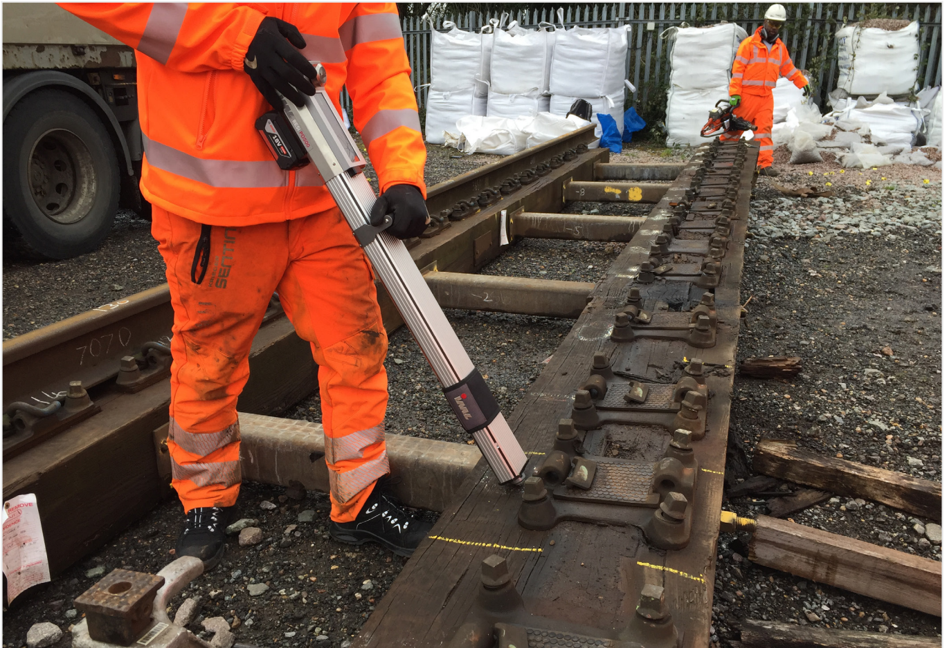
Figure 1: The IML Resi-PD 500 in use on longitudinal bearers removed from track following the derailment at Wanstead Park.
