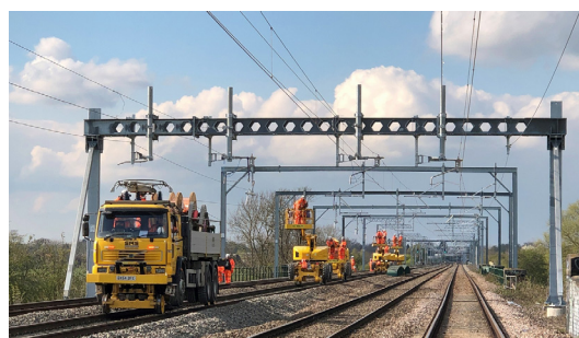
RRV plant undertaking construction on Midland Main Line
