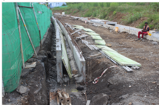
Figure 3: Water courses being constructed either side of the route.
