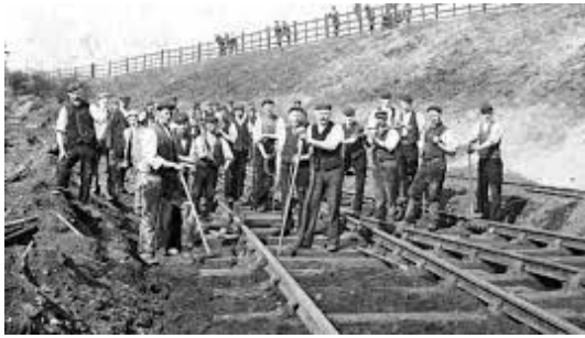
Laying track Ryecroft late 19th Century
