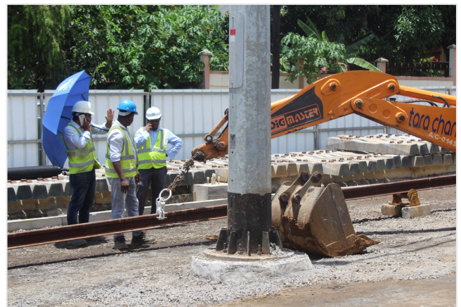
Figure 6: Rails being initially positioned using rollers and a digger arm.
