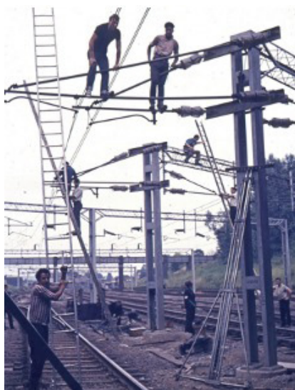
Mk1 OLE Installation Kenton 1964
