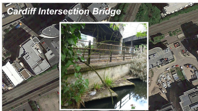
Figure 3: Cardiff Intersection Bridge - Cardiff Central Station approach, Wales and Western Route.
