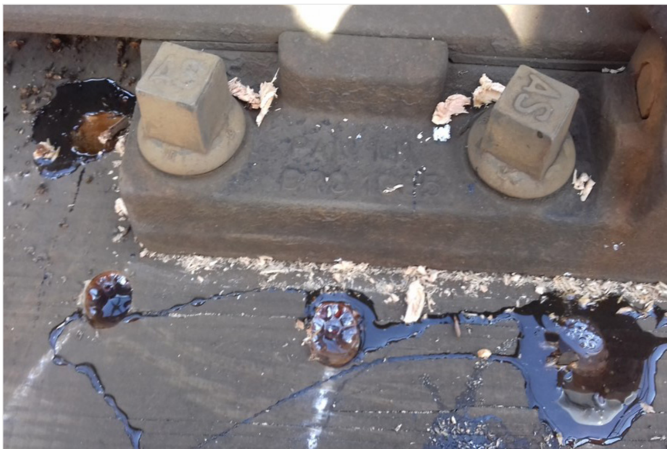
Figure 5: A boron based preservative gel installed into a longitudinal bearer in situ (actual hole size and spacing exaggerated for illustrative purposes and must not be used as a basis for undertaking treatment). Photo - Dr John Williams.
