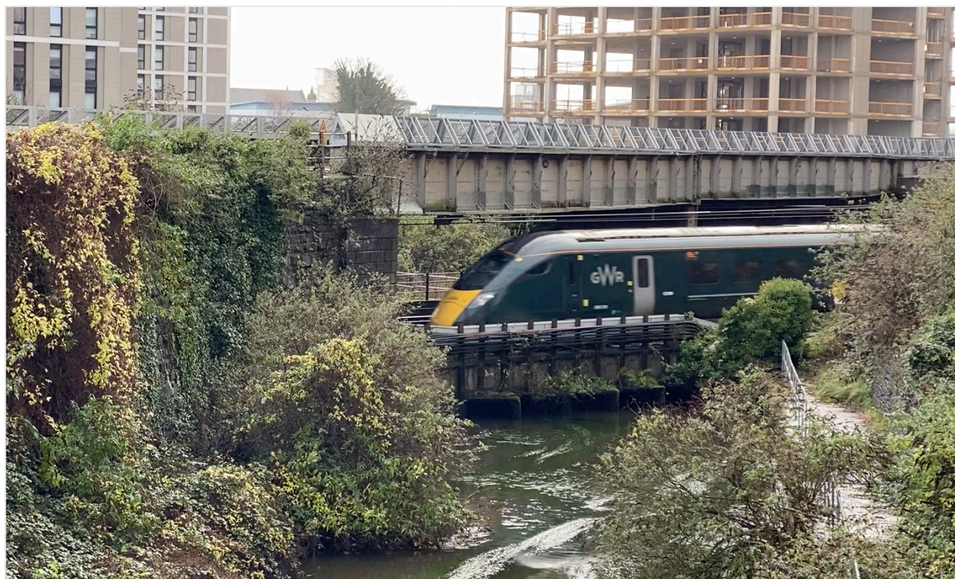
Figure 14: Class 800 (IET) travelling 'under the wires' at Cardiff Intersection Bridge.
