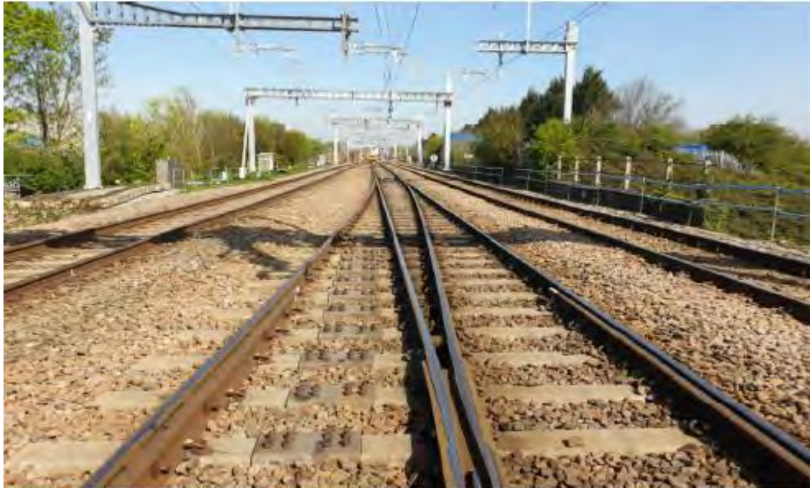
GENERAL VIEW OF POINTS 8743, SHOWING PART OF THE BRIDGE AND CROSSOVER 3744 IN BACKGROUND (LOOKING NORTH)
