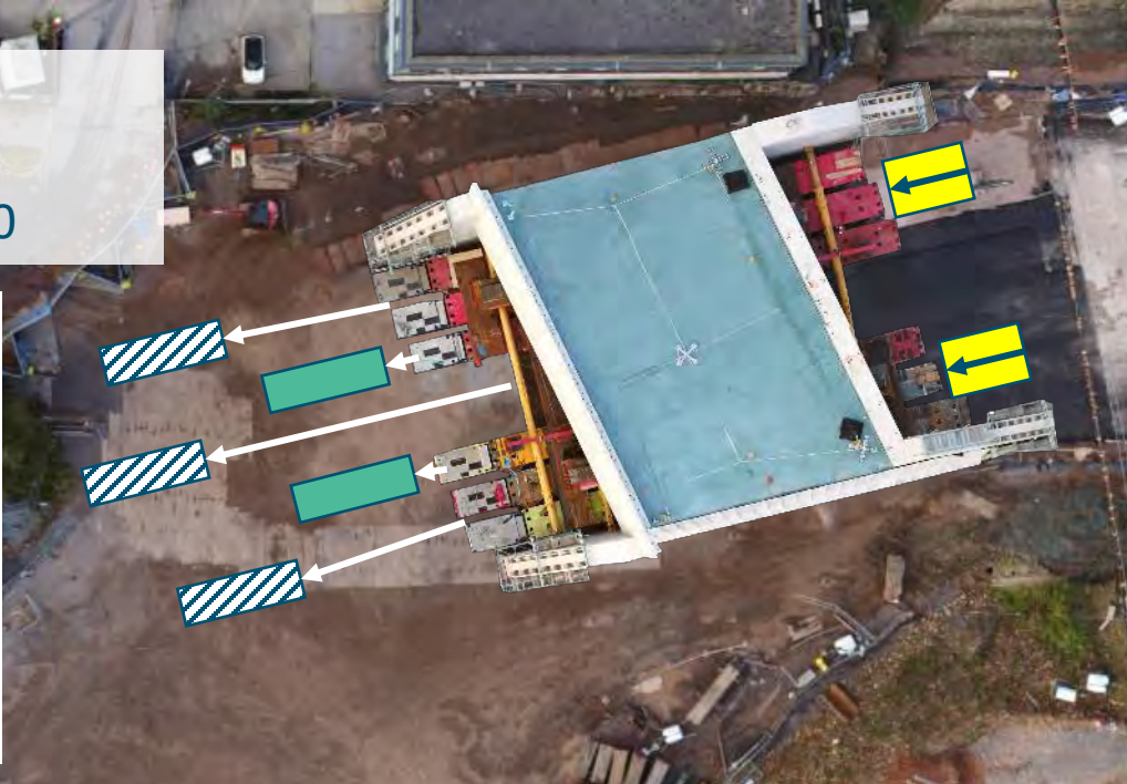
Pushing using dozers
