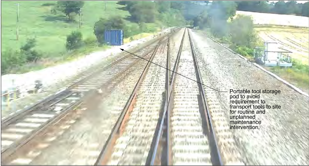
- Extract from Civils Design Drawing Showing Provision of Portable Tool Storage Pod and Safe Walkway
