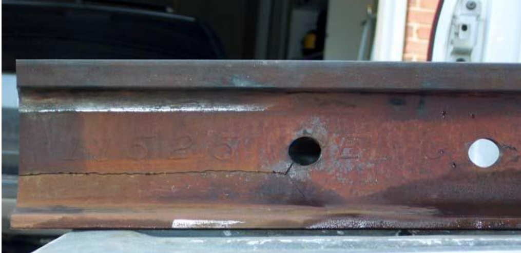
Figure 3.21 Bolt Hole Failure (courtesy AREMA)
