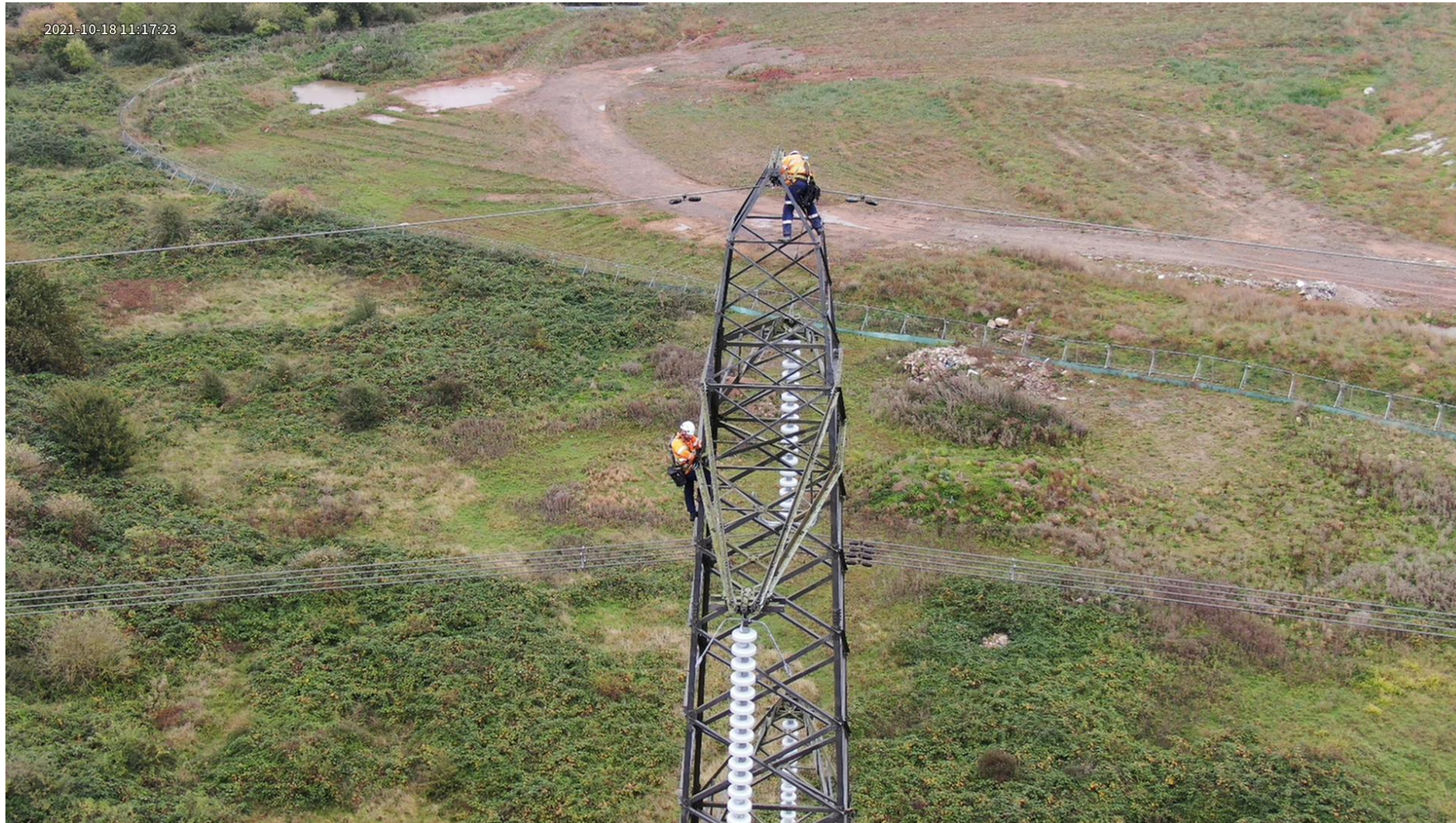
Video showing Western Power repairing a neutral section supplying a NR 25000v substations following a major storm
