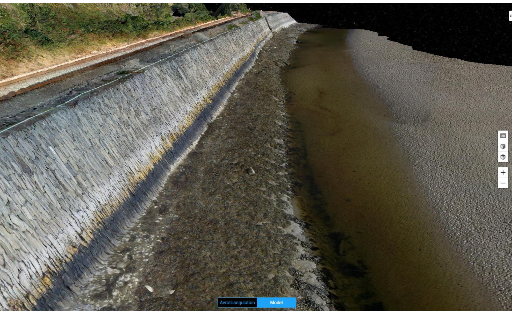
3D Image Created in North Wales During a Sea Wall Defence Inspection, (this image has over 200 pictures stitched together)
