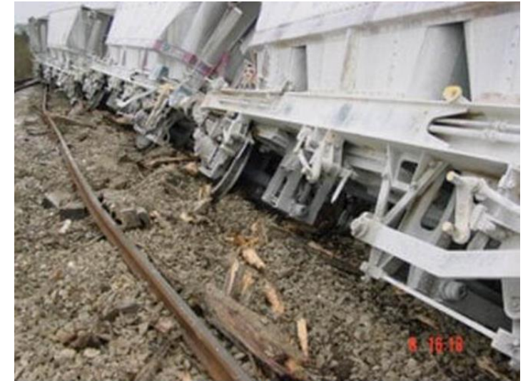
Pontsmill Derailment Picture 4 Copyright Stephen Heginbotham Railcoach
