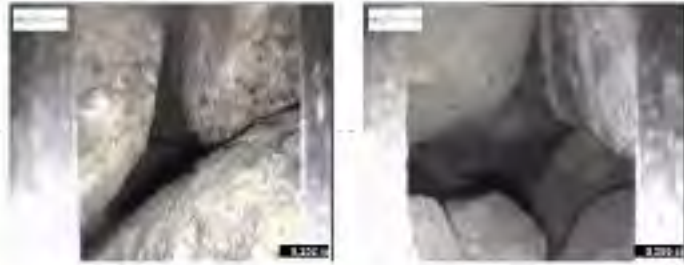
Clean Ballast depth
