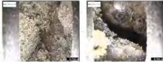
Fouled Ballast depth (dust / fines generated from tamping)
