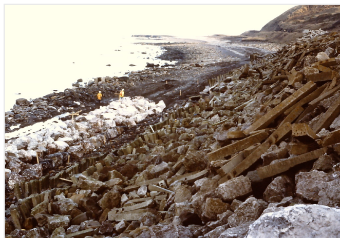
Figure 14: Construction of rock bund at Micklam.
