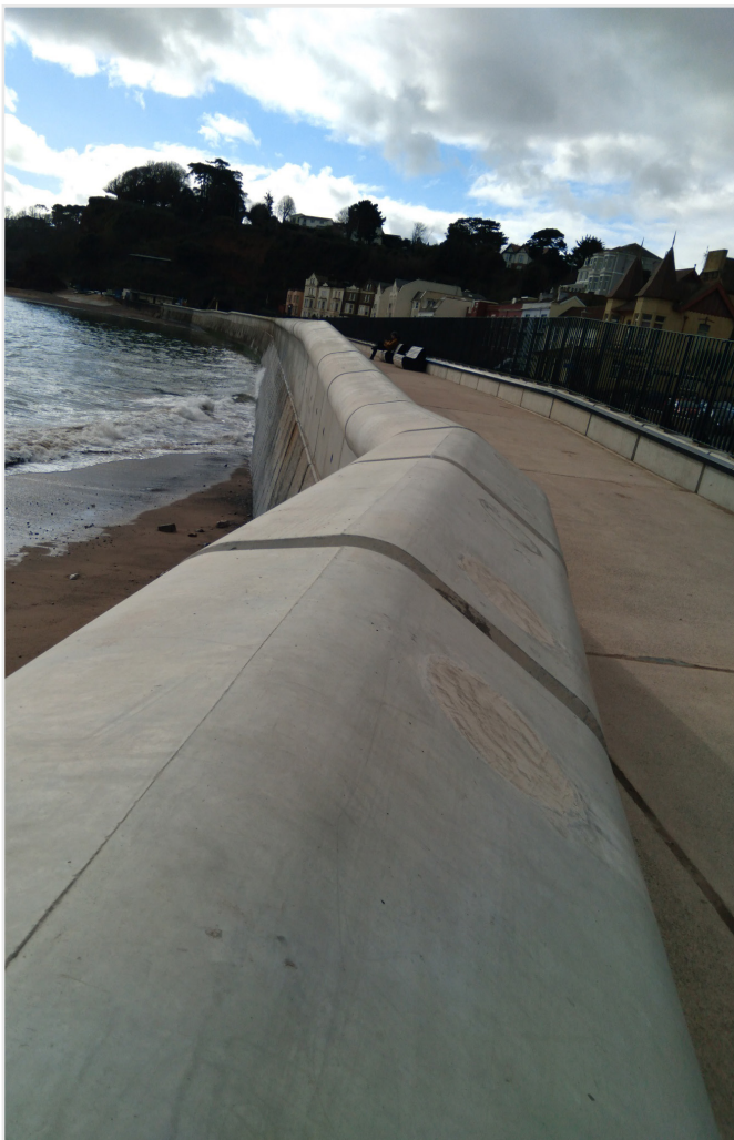
Figure 9: Reconstructed sea wall at Dawlish.
