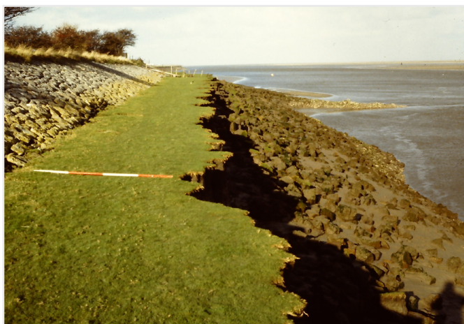
Figure 13: Lord Vivian's Embankment.
