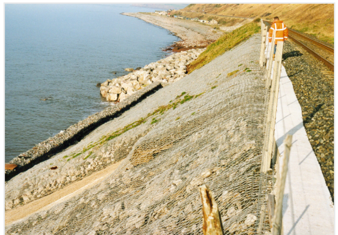
Figure 16: Upper slope with 6G stone and rock netting at Nethertown.
