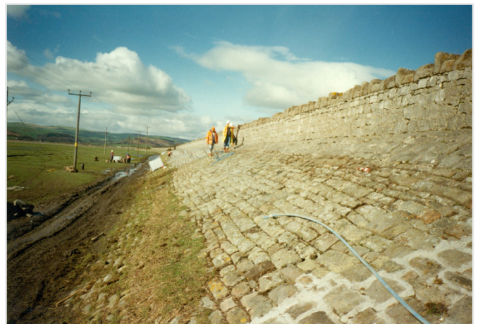
Figure 2: Revetment at Capes Head embankment.
