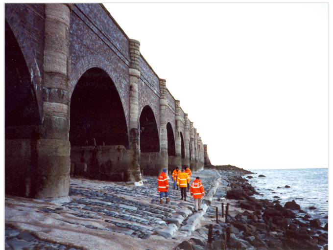
Figure 8: Viaduct at Llanfairfechan.
