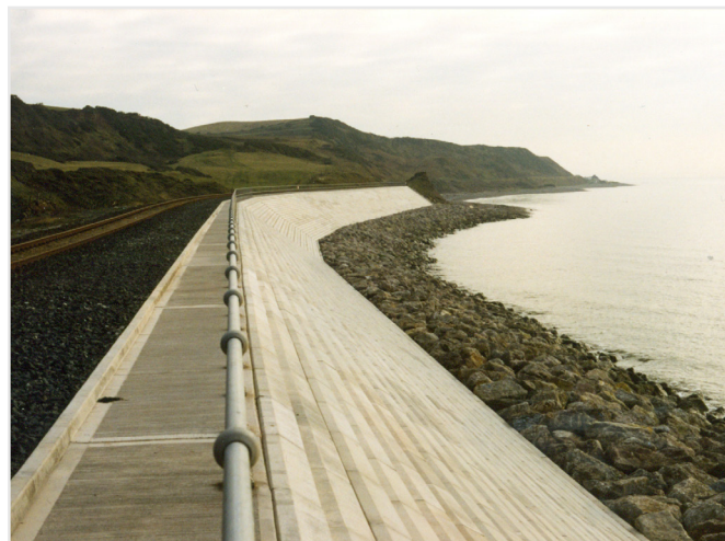
Figure 12: Upgraded sea defences at St. Bees.
