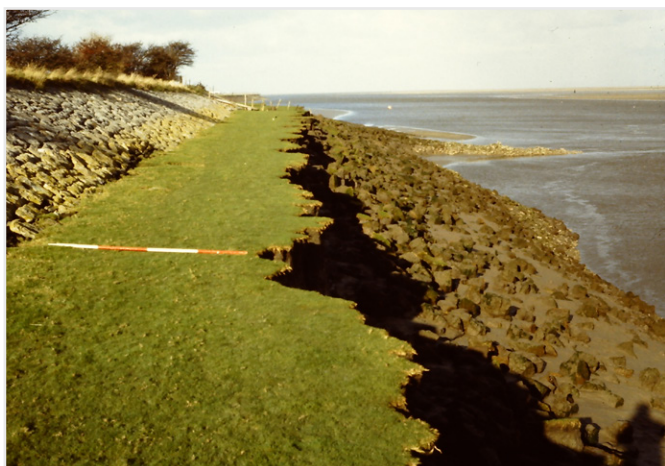
Figure 13: Lord Vivian's Embankment.
