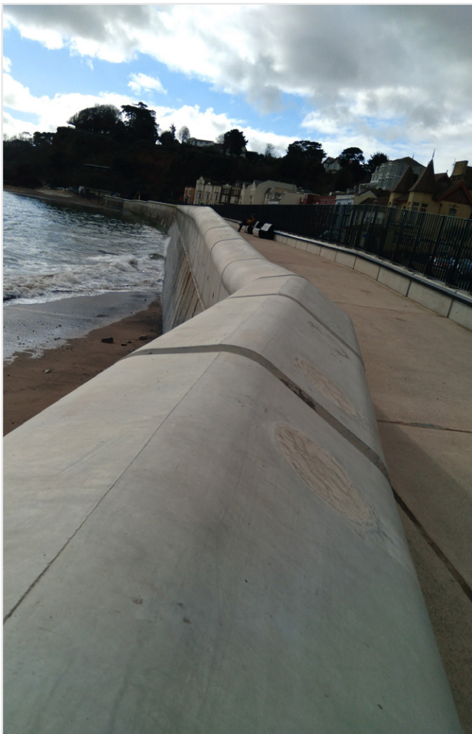
Figure 9: Reconstructed sea wall at Dawlish.
