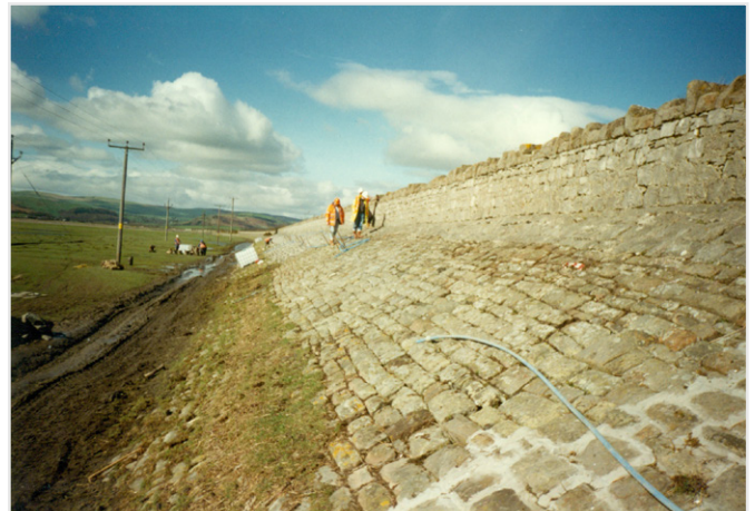
Figure 2: Revetment at Capes Head embankment.
