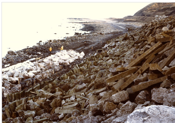
Figure 14: Construction of rock bund at Micklam.
