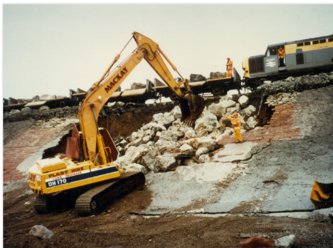
Figure 11: Repairs to the sea wall at St. Bees.
