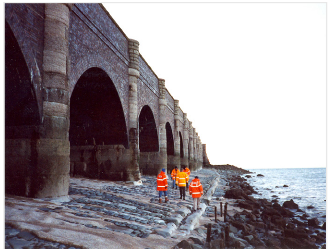
Figure 8: Viaduct at Llanfairfechan.
