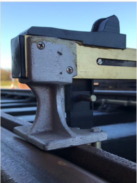
Figure 12: Track gauge foot registering only on switch rail.
