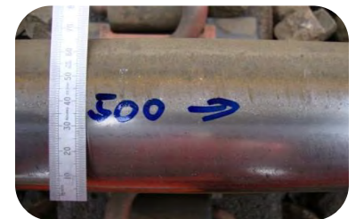
HP335 – no cracks (3 months after grinding)
