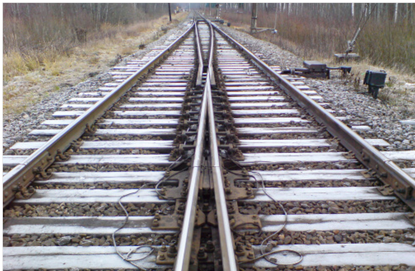
Figure 6: A swing nose crossing. Photo Wikimedia/Dzelcēļnieks, CC-SA4 licence
