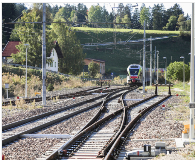
Figure 10: Trap points at the end of a siding or loop line joining a main line. Photo Wikimedia/Falk2, CC-SA4 licence.
