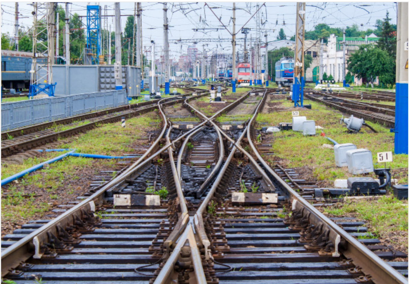
Figure 9: A double (internal) slip crossover, where a train approaching from any direction can either go straight on or take the diverging route. There are eight movable switch rails in this layout, all of which must be moved, detected and locked (Photo Shutterstock/ Leonid Andronov).
