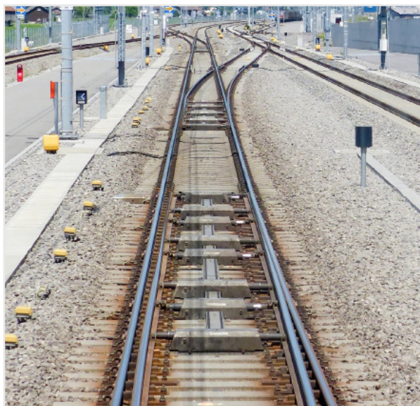
Figure 4: (Above left) Multiple operating mechanisms in use on a high-speed turnout. In this example there is just one machine driving the points (to the left of the switch tips), and the power from it is transmitted hydraulically to several setting and locking mechanisms along the length of the switch rails (Photo Francis How).
