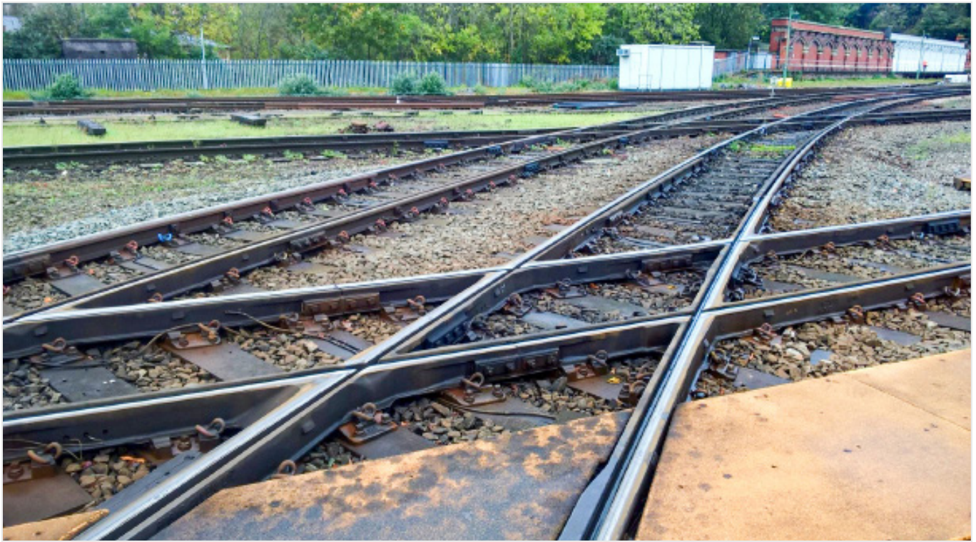
Figure 7: A fixed diamond crossing. A train on either track can only go straight on, not diverge (Photo Network Rail).
