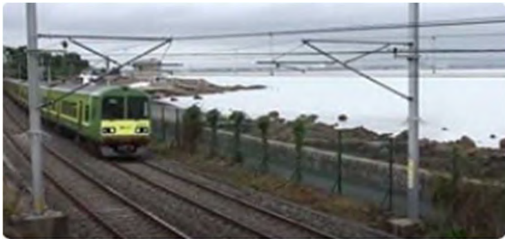
40km of Overhead Electrification & 12 new substations
