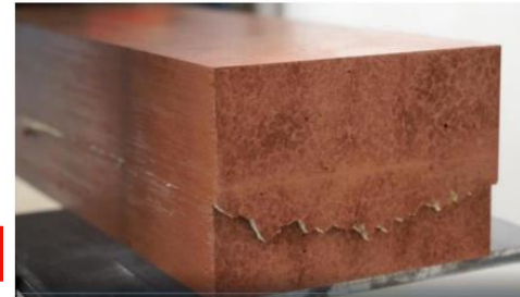
Figure 1: Delamination of FFU material
