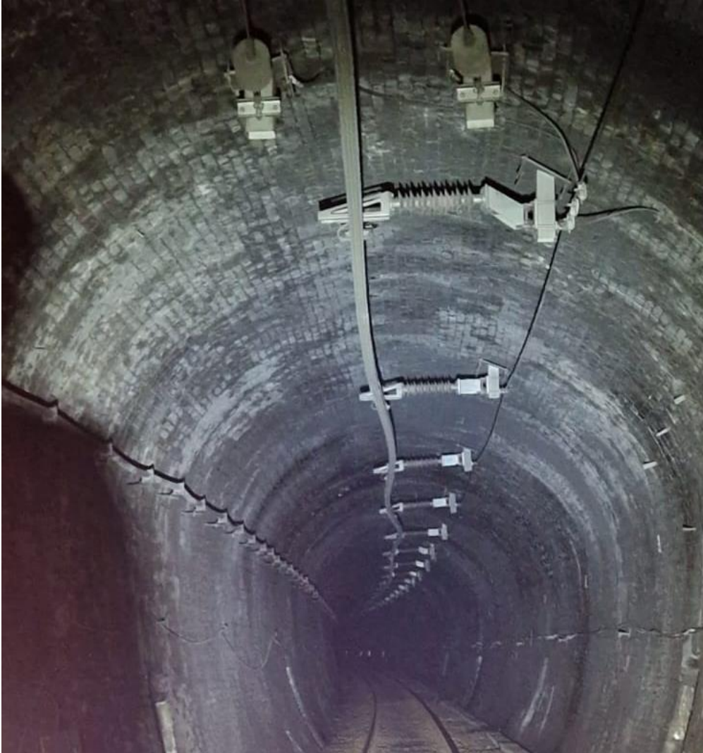
Conductor beam misalignment – June 2023
