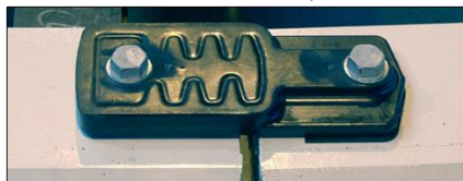
Elastic coupling for concrete sleeper with through bolt connection (Swt 7)
