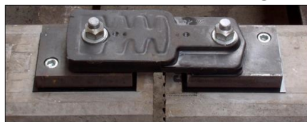
Elastic coupling with adapter plate for concrete sleeper with dowel fastening (Swt 13)
