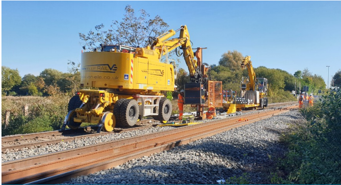
Figure 8: Trackbed stabilisation with micro-piling and site condition at Case Study 1, Van Elle Ltd
