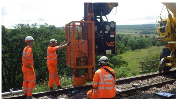
Figure 10b: Case Study 4 pile installation.
