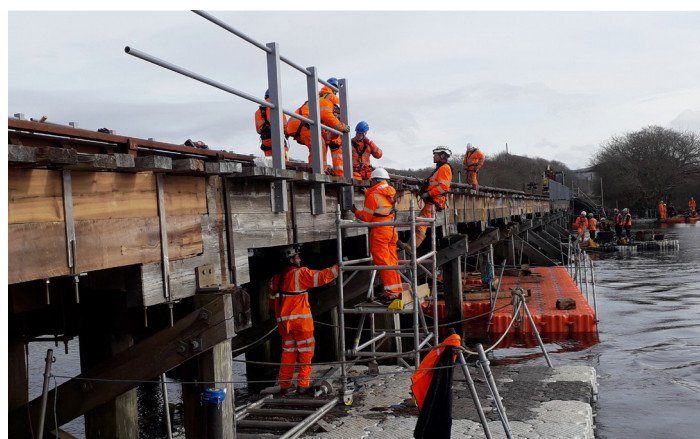
Figure 11: Staff working from cellular pontoons and tethered with safety lines
