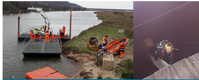
Figure 15: Barge and pontoons. Diver navigating a trestle outrigger
