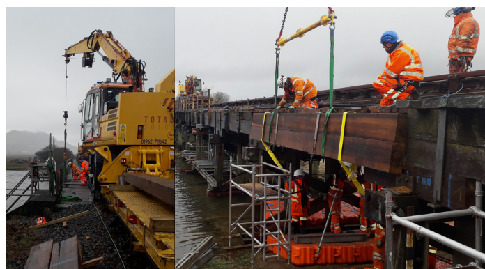
Figure 12: RRV delivering materials and Edgebeams being replaced by RRV (staff tethered with safety lines)
