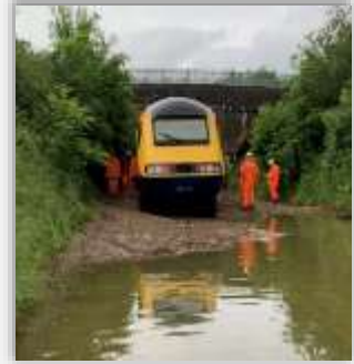
Track flooding and wash-out incident at Pen Green, Corby 2022
