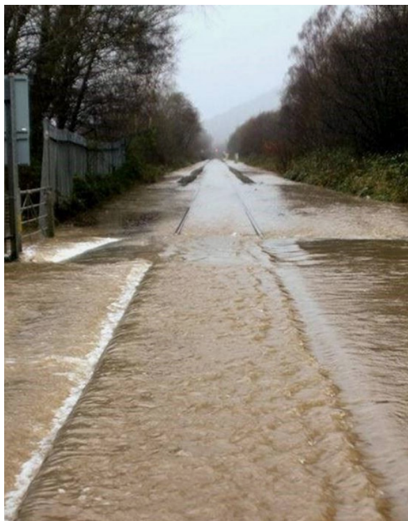
Figure 5: Flooding at Cwmbach, a regular occurrence after adverse weather
