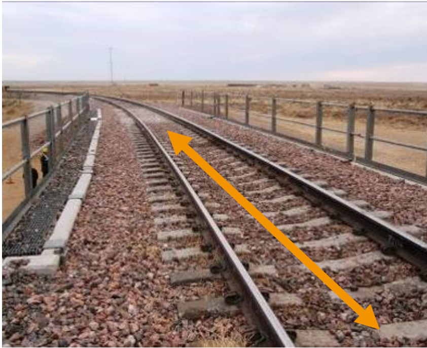
Section with under ballast mat in perfect condition
