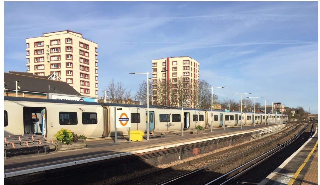
Norwood Junction, 203m DF Platform (above) Norwood Junction, 184m UF Platform
