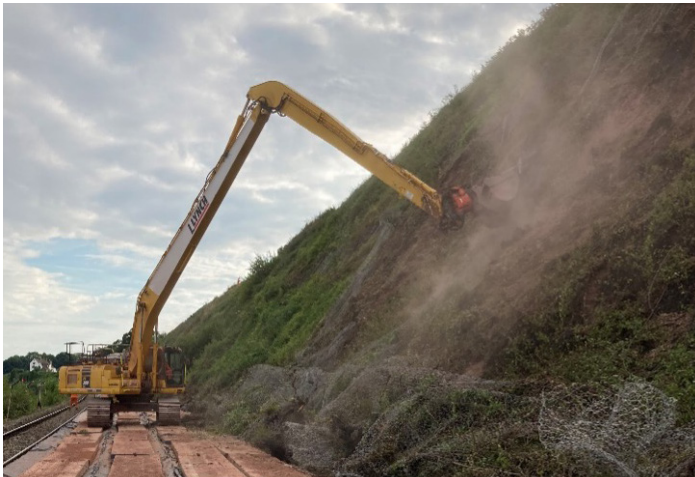
Figure 3: Long reach excavator regrading topsoil from cutting face under NRDD guidance
