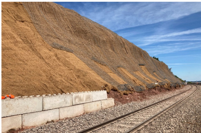
Figure 5: Regraded slope with coir erosion control matting installed as well as partly installed galvanised steel mesh
