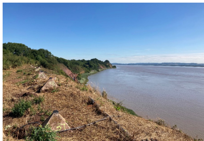
Figure 6: Picture of Severn Estuary from top of the cutting overlooking the worksite
