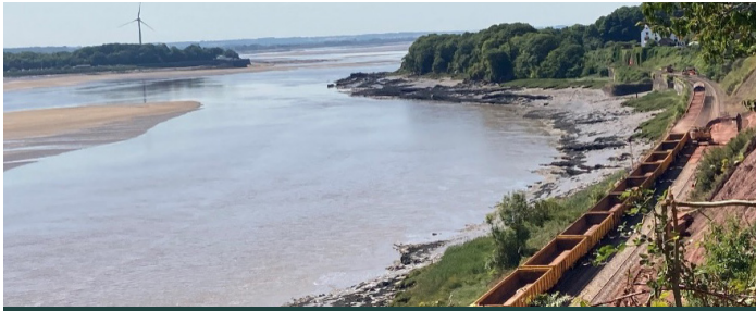
Figure 2: Engineering Train stationary on site location while wagons are being loaded by excavators
