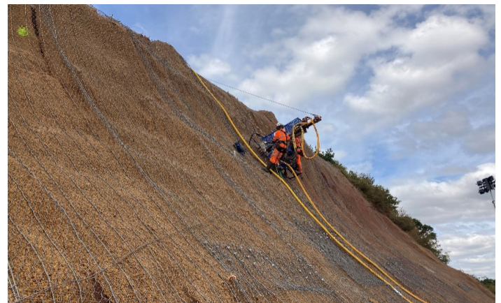
Figure 4: Rope trained operative drilling into cutting face using a suspended drilling rig from the top of the cutting.
