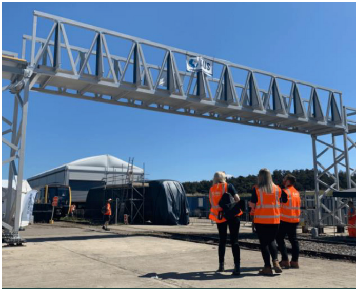
Figure 8: Partially Completed Test Footbridge at Rail Live 2021
