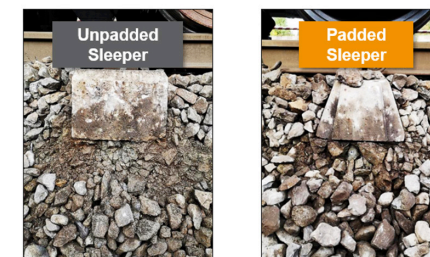
Figure 7 Benefits of using under-sleeper pads for loading and reduced ballast attrition. (photos courtesy A Moore)
