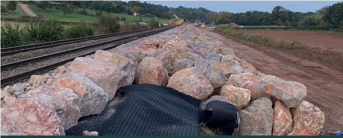
Figure 6: Image of rocks being placed on top of matting.
