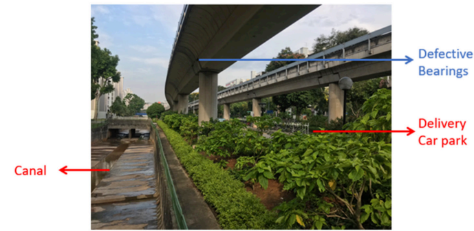
Figure 1: Site Conditions and Constraint for Pier CN0683.
