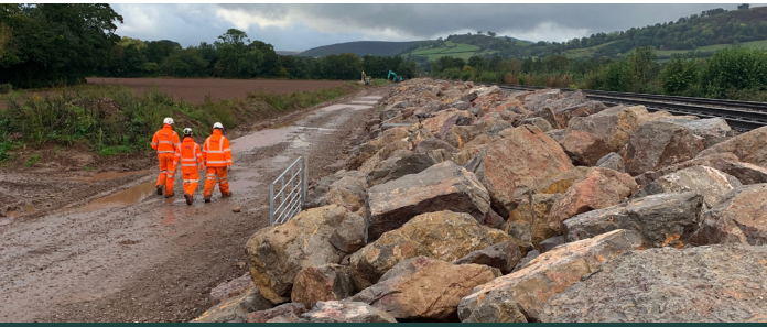
Figure 9: Restoration of site.
