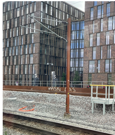
Figure 6: Danish electrification mast.
