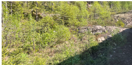
Figure 8: Norwegian lineside verge cleared of large trees.
