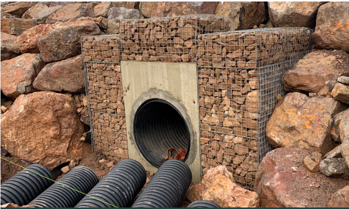
Figure 7: Drainage improvements, including increased outfall capacity and gabion baskets.
