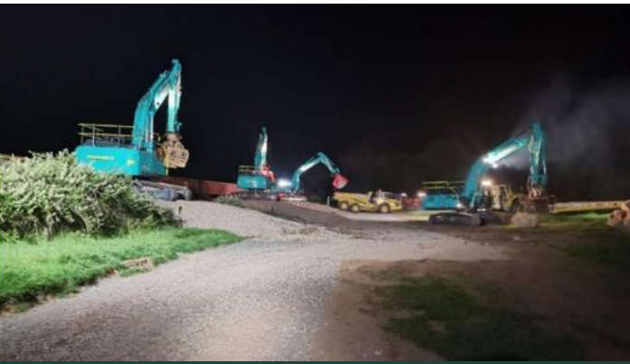
Figure 8: Rock armour being delivered by rail.
