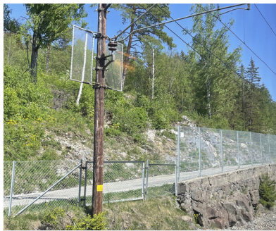
Figure 4: Legacy timber electrification mast.
