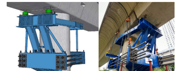
Figure 4: Friction Clamping System Design (Left) and On Site (Right). (Photos from PSC Freyssinet (Singapore) Pte Ltd)
