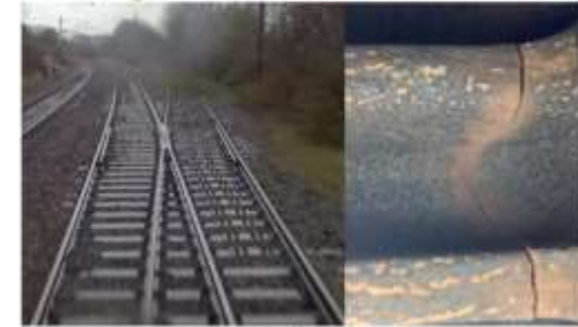
Example of a break at a Tin Metal weld
