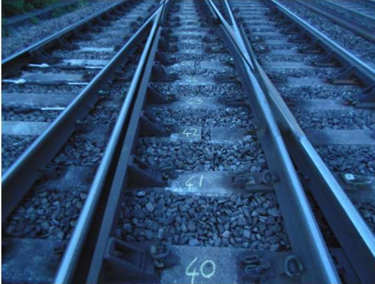
BH49 Pts – Emergency Gauge Tie Bars fitted on Up Fast Line in crossing area
