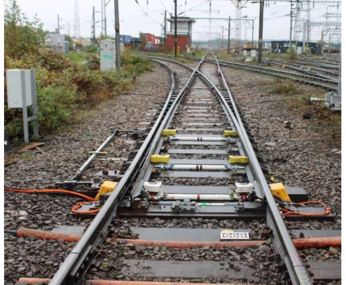
NH66B Pts – Completed POE Conversion
