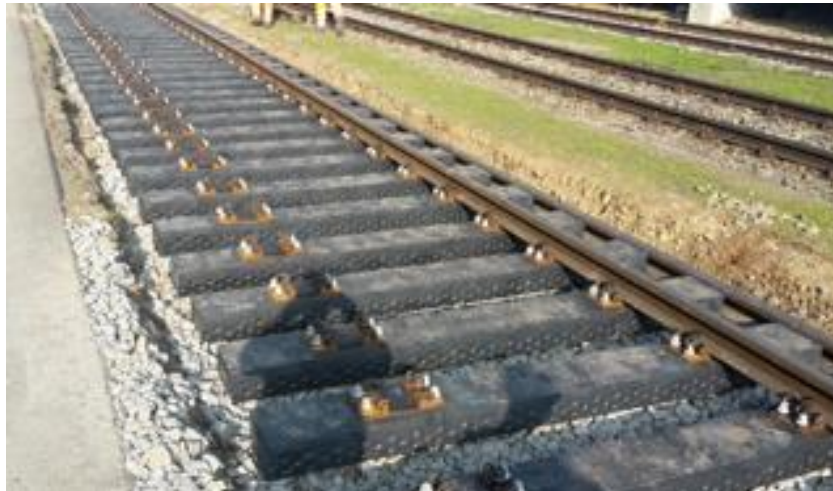
Baseplated Plastic Recycled Composite \approx 36\text{kgco}^2\text{e}
