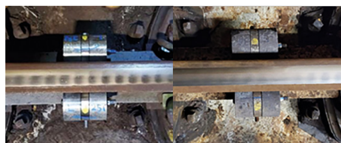
Figure 12: Rail Roughness immediately after damper installation - four months after grinding (Left) and one year after damper installation - four months after grinding (Right).
