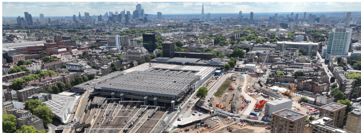
Aerial view of HS2's London Euston Station site (Image courtesy of www.hs2.org.uk media centre).
