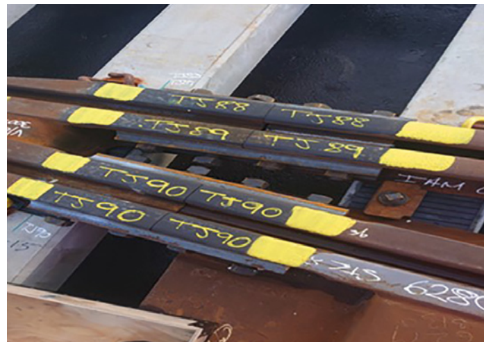
Figure 8: Close proximity of bolts warranted interlacing and head to tail reverse assembly and, in some cases, the adoption of flat fishplate profiles. (Image courtesy of Progress Rail).
