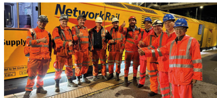
Figure 4: CHKRI MTR team on a night shift at Leeds watching track repairs carried out on the mobile maintenance train. (Photo courtesy of K. Ting).
