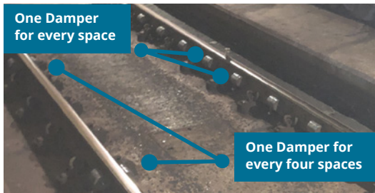
Figure 6: Installation of RCTMD on Testing Rails.
