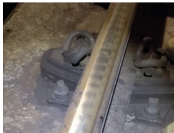
Figure 5: Corrugation of Test Rail.
