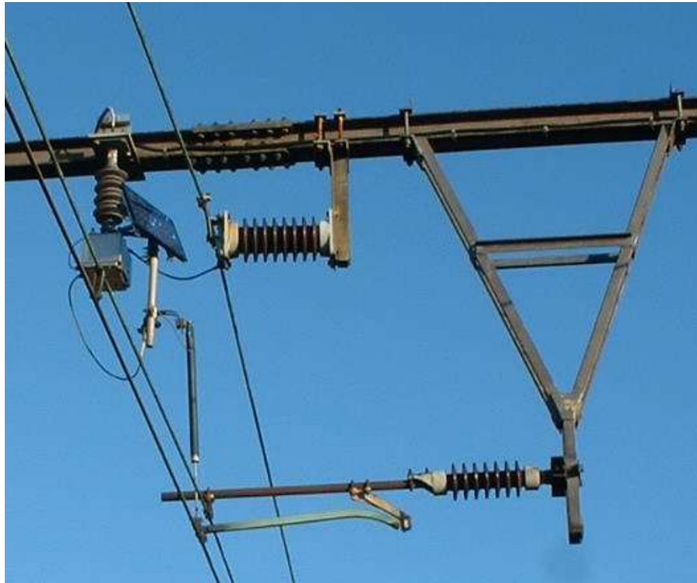
Panchex at Chadwell Heath (courtesy of PWI)
