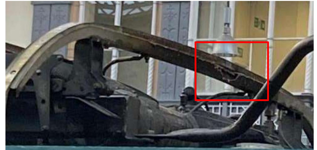
Ice damaged pantograph - 2023
