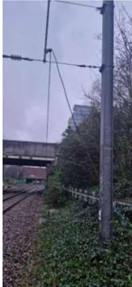
Examples of earth wire failures
